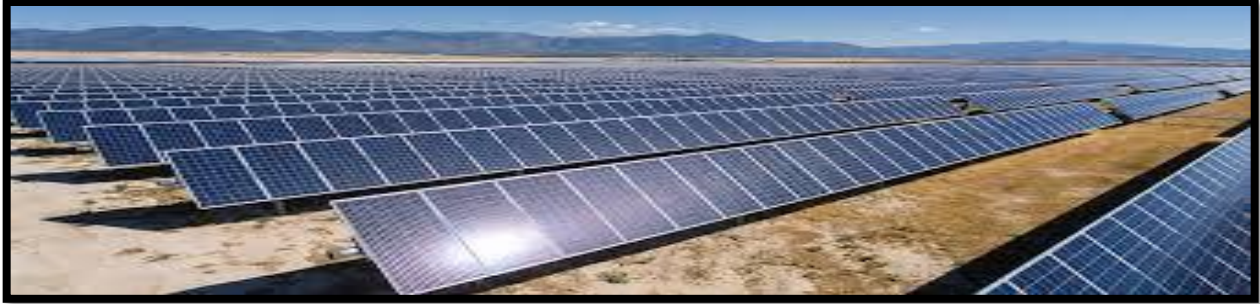
PICTURE 3. SOURCE: UTAH SOLAR WORKS
