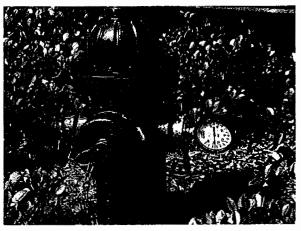
On-site Fire System Pressure Reading 135 PSI Hydrant was flushed prior to reading.
