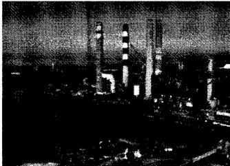
The station operates four (4) pulverized coal-fired steam units equipped with desulfurization scrubbers and electrostatic precipitators. The station's coal-fired units have recently undergone the addition of air pollution control systems called Selective Catalytic Reduction (SCR). The SCR installations occurred from 2007 to the spring of 2010. In addition, the station operates one (1) aero-derivative combustion turbine that entered into service in
