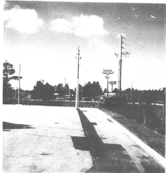
(RD-7b) HOLIDAY INN PARKING LOT LOOKING TOWARDS AIRPORT ROAD. JEA'S NEW UNDERGROUND INSTALLED IN CUT PAVEMENT. DISTANCE FROM POLE TO FIRST MANHOLE 190 FEET
