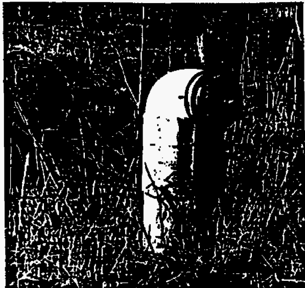
Figure B-5-1(a) Dry hydrant.
