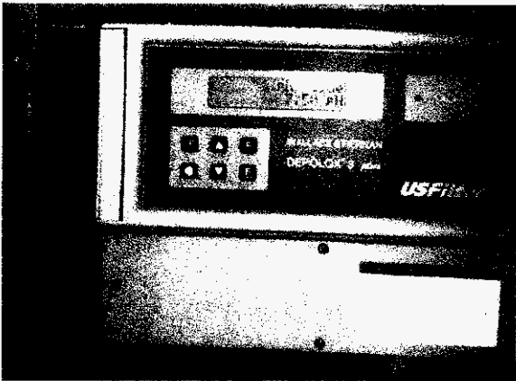
Each plant has automatic pH and Chlorine readers.
