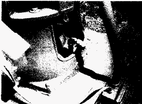
Cracks noted in the seal around the well head at Well 4 have been nicely corrected since the last sanitary survey.
