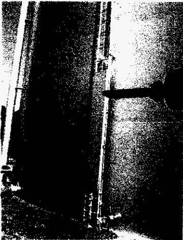
Wayne ground storage tank with ladder guard.
