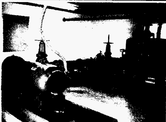
High service pumps at Wayne tank - note one is auxiliary pump.
