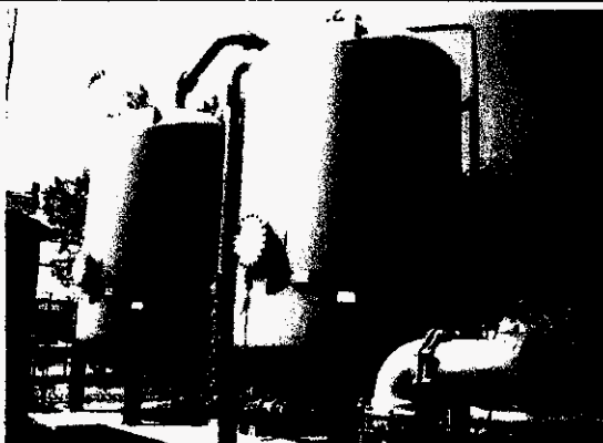
GAC filters are located at Wells 3 and 8. These at Well 8 were recently painted.
