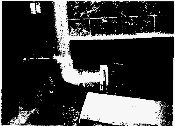
Overflow from Gulf Beach ground storage tank.
