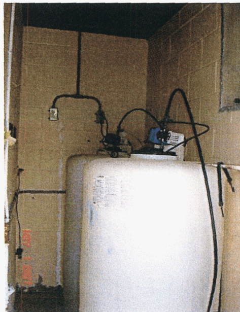
Sodium Hypochlorite tanks.
