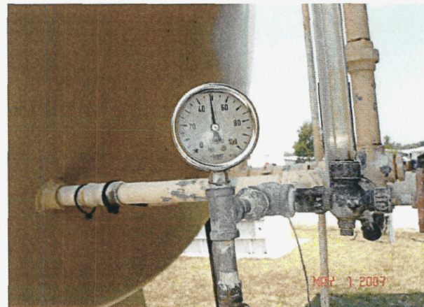
Static distribution system pressure, 49 psi, (no pumps running.)
