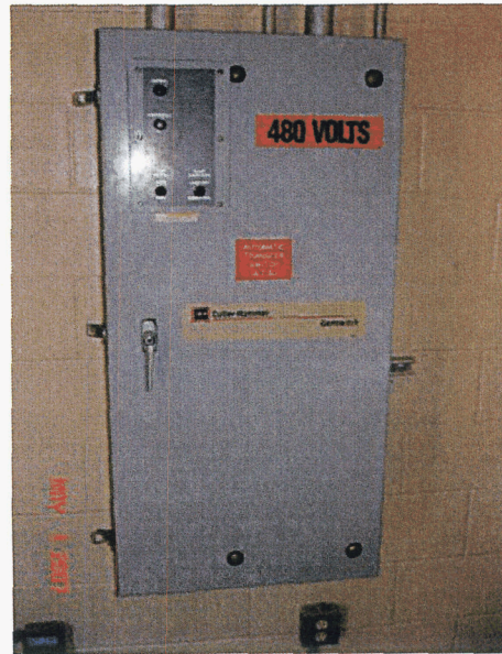
Emergency generator transfer switch.
