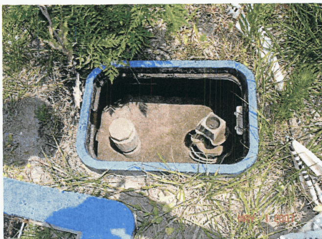
In-ground Eclipse Blow-off assembly
