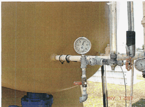
Well #1 running, water pressure at 56 psi .
