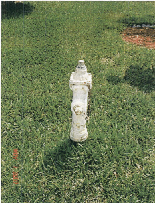
Above ground Kupferle, 2-inch blow-off.
