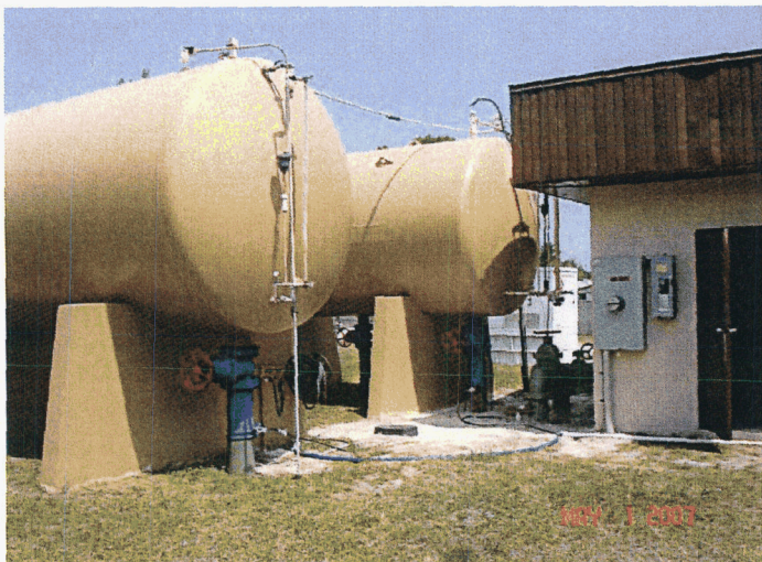
Pump and Chlorine building, and pressure equalization/storage tanks at Water Facility.
