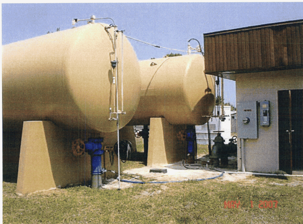
Sodium Hypochlorite supply lines on ground, split and connecting to Tank #1 and #2 distribution piping.
