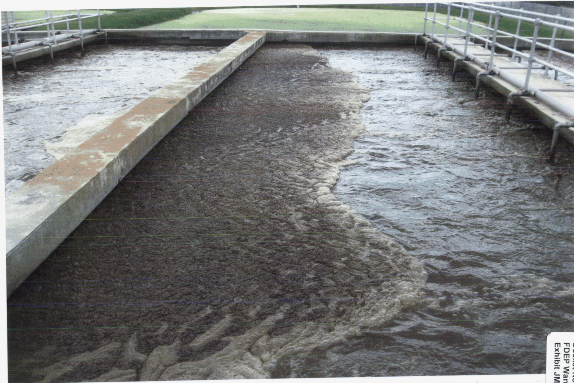
Photo above of the MLSS in the aeration tanks
