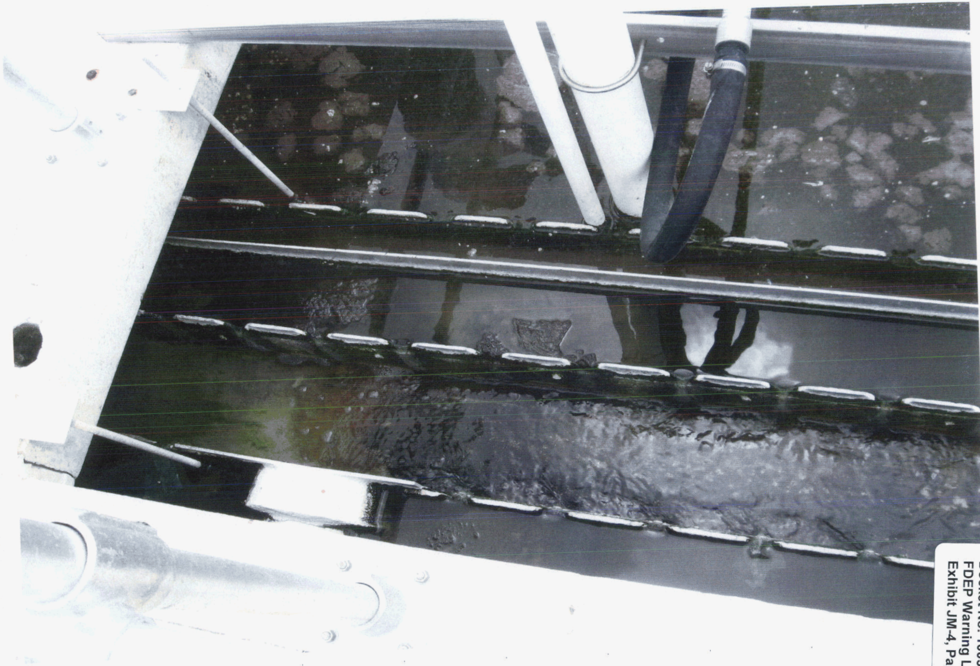
Photo above of the northern clarifier's weir
