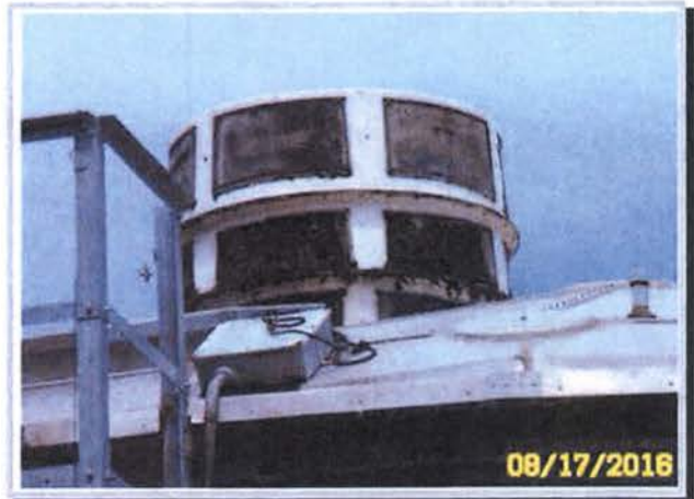
Aerator at Tank 1 Well 2 - 316,000 gal tank.
