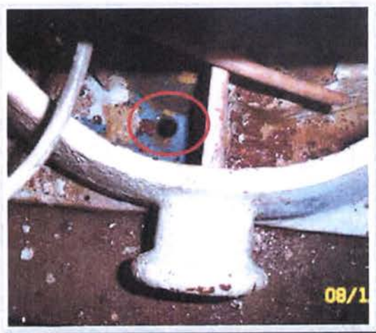
Well 2 at office. Improper well casing vent.
