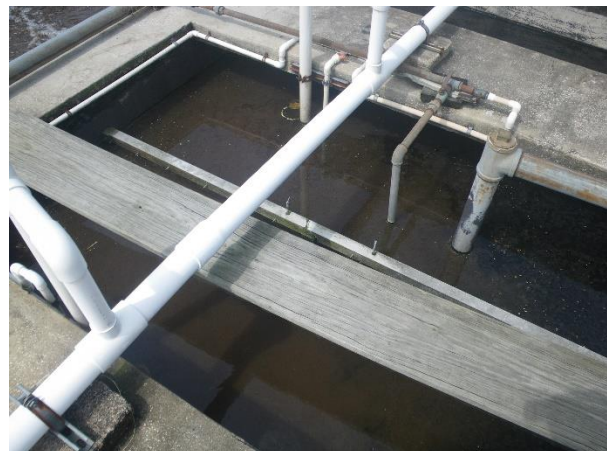
6 Clarifier with solids in the water column
