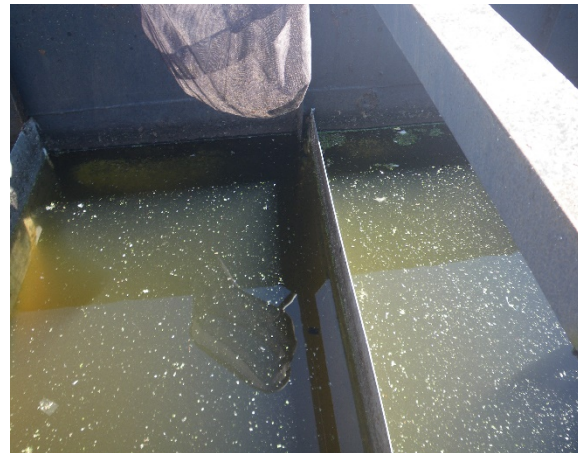
16 Separated baffle in CCC
