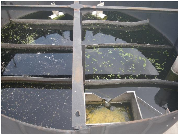
9 Chlorine contact chamber
