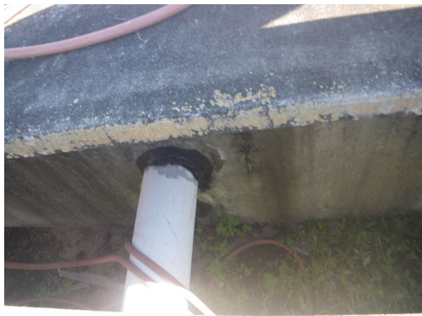
12 Leak around pipe connection
