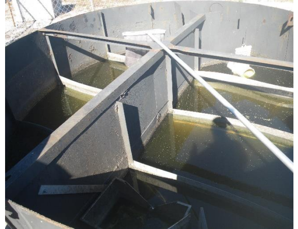
14 Chlorine contact chamber
