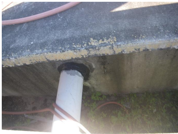
12 Leak around pipe connection
