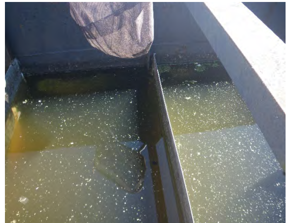
16 Separated baffle in CCC
