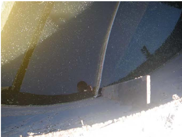
15 Separated baffle in CCC
