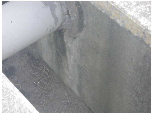
8 Leak on wall of plant
