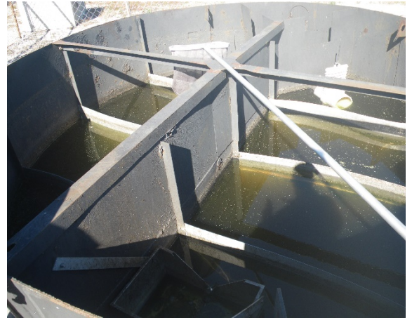
14 Chlorine contact chamber
