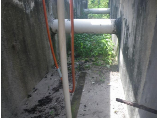
13 Leak from connection pipe
