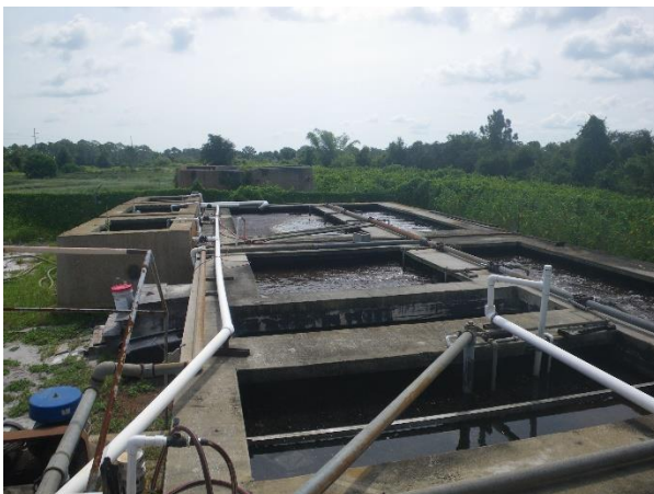
5 Aeration basins, clarifiers, and digesters
