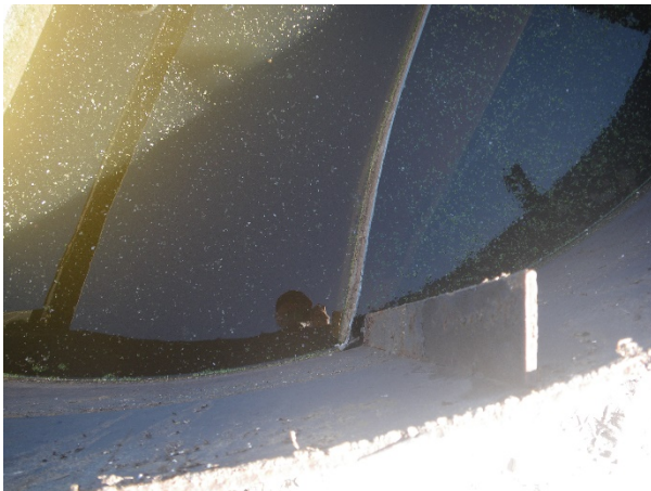
15 Separated baffle in CCC
