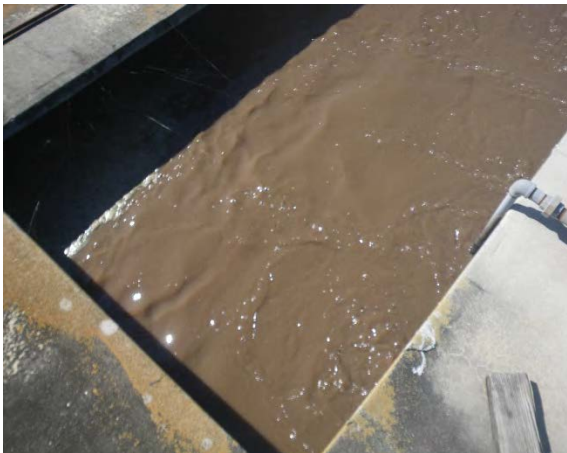
9 Dead spot at diffuser in third basin
