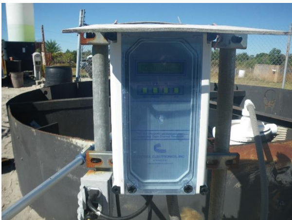
17 Ultrasonic flow meter
