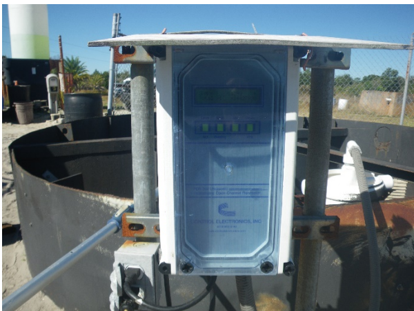
17 Ultrasonic flow meter
