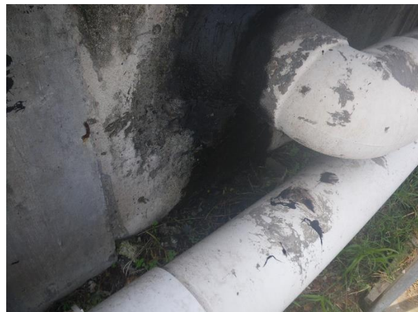
12 Leak from connection pipe
