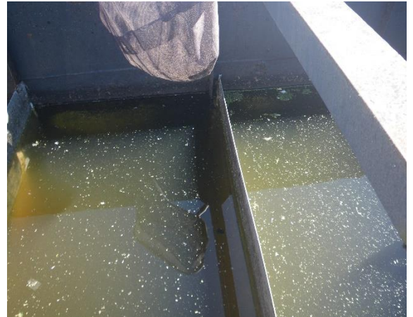
16 Separated baffle in CCC
