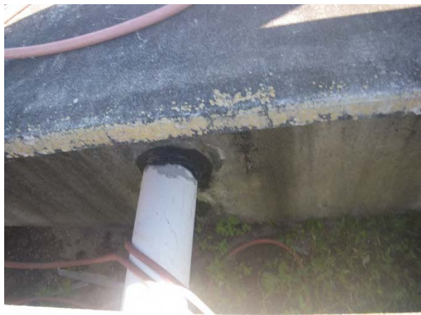
12 Leak around pipe connection
