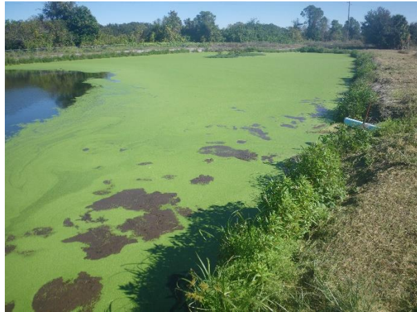
2 Sludge in percolation pond
