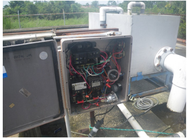
2 Elapsed time meters placed at surge tank
