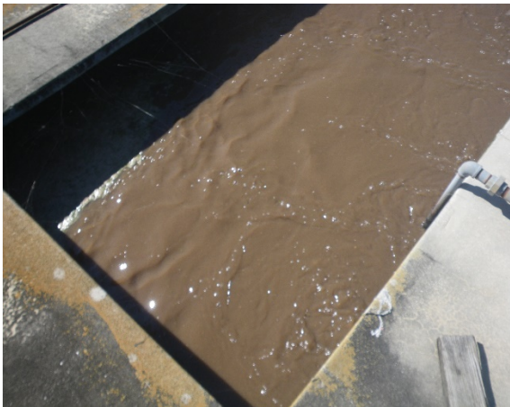
9 Dead spot at diffuser in third basin
