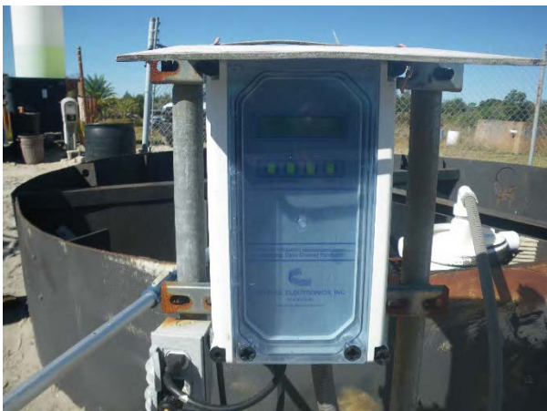
17 Ultrasonic flow meter
