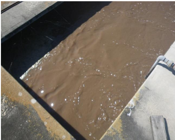
9 Dead spot at diffuser in third basin
