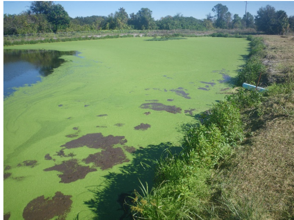
2 Sludge in percolation pond
