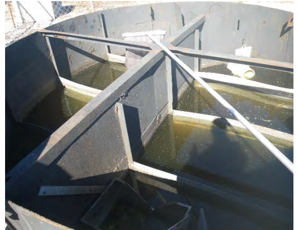
14 Chlorine contact chamber
