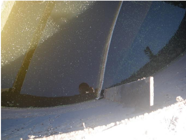
15 Separated baffle in CCC
