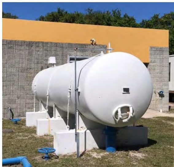
Figure 2-13: Hydropneumatic Tank
