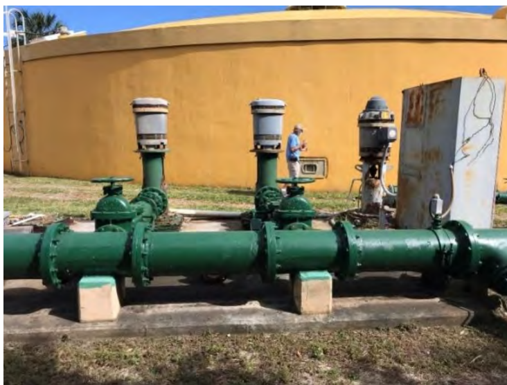
Figure 2-11: Fire and Irrigation Pumps
