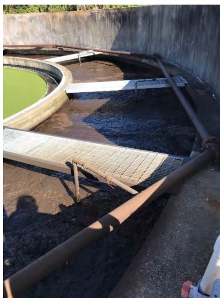
Figure 2-2: Extended Aeration Basin
