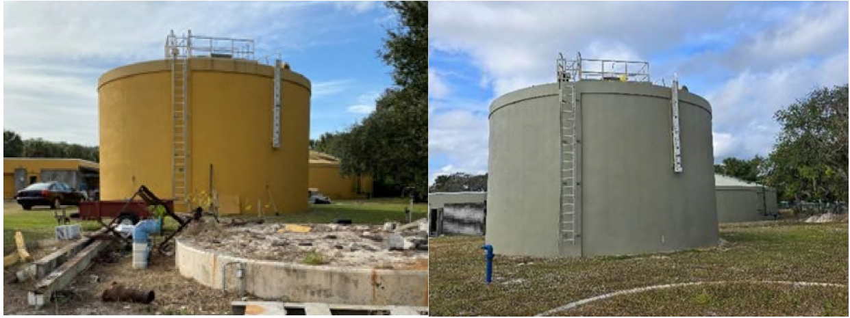
Before (Left) & After (Right): Ground Storage Tank Recoating and debris removal.
