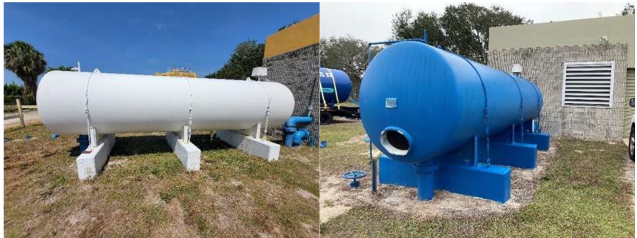
Before (Left) & After (Right): Ground Storage Tank Recoating and debris removal.
