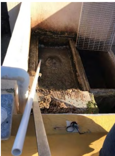
Figure 2-1: Headworks Influent Screen
