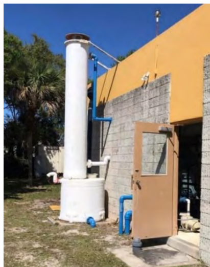
Figure 2-6: Aeration Tower and Clearwell
