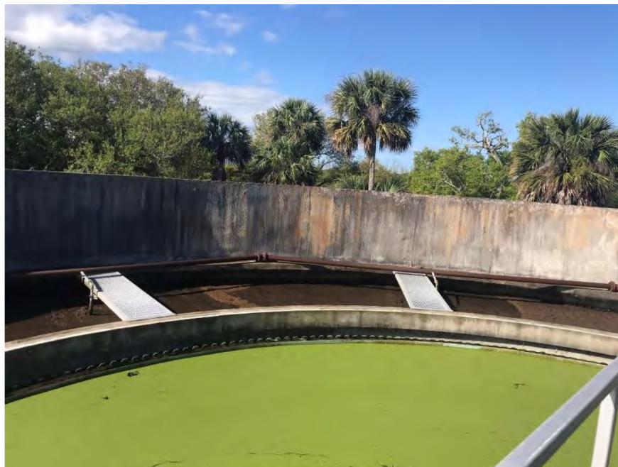
Figure 2-11: Clarifier Weir and Launder
