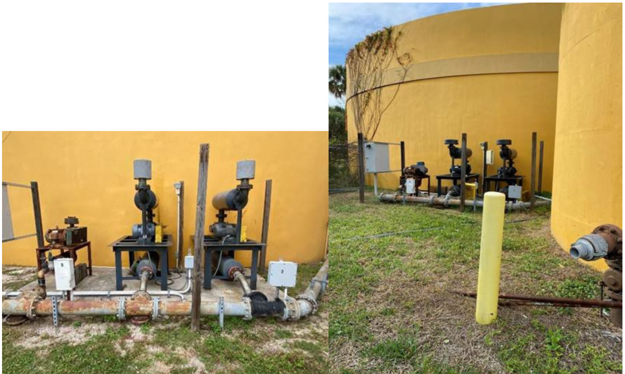
Before: Rusted piping and blower motors.
