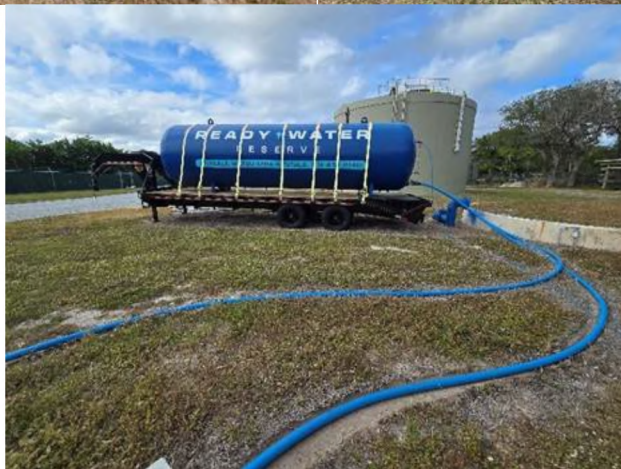
Before (Left) & After (Right/Bottom): Hydro tank leaks discovered during interior recoating requiring tank replacement, temporary tank in place until new tank can be designed and installed.
