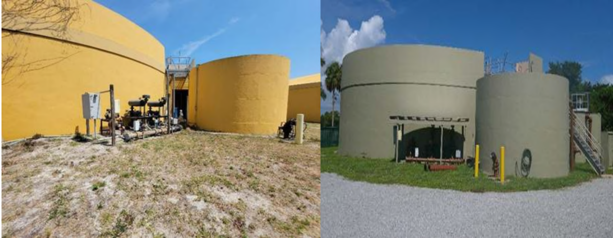
Before (Left) & After (Right): Tank recoating and shade structure for blowers (Access Road also visible).
