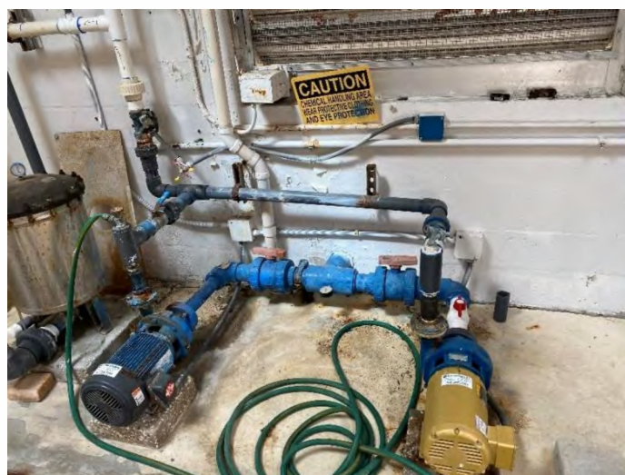
Figure 2-8: Well #2 Booster Pumps
