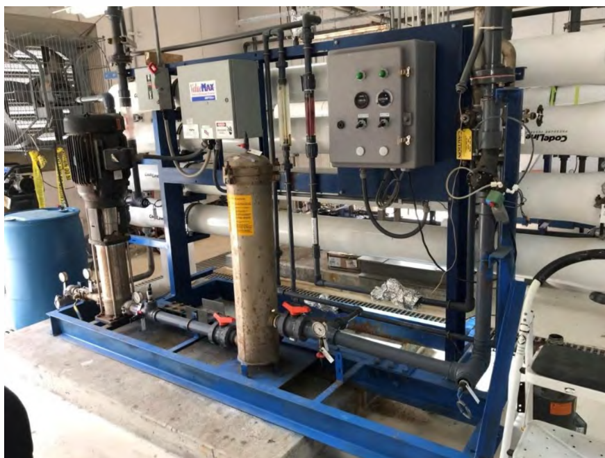
Figure 2-4: ValueMax RO System
