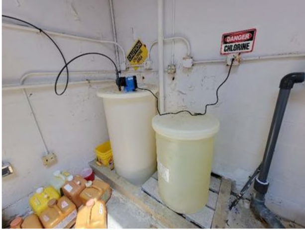
Before (Left) & After (Right): Chemical containment inadequate (note dry chemicals all over floor in before photo).
