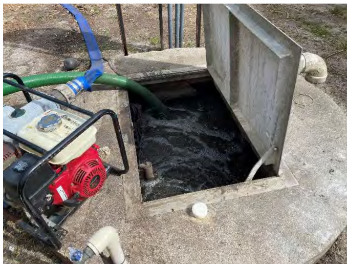
Figure 2-10: Onsite Pump Station and Temporary Pump
