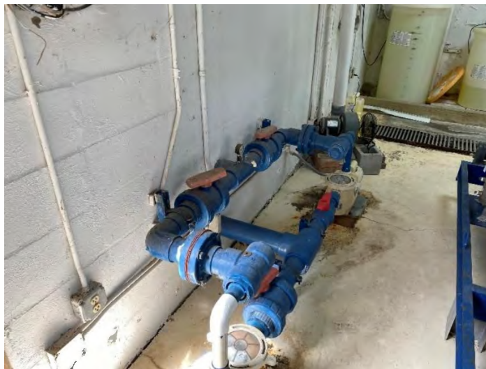
Figure 2-9: Transfer Pumps
