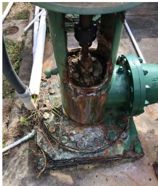
Figure 2-18: Fire and Irrigation Pump Condition
