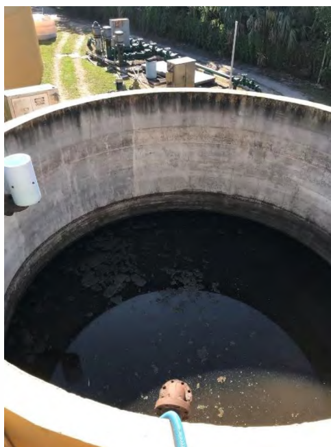
Figure 2-6: Sludge Holding Tank
