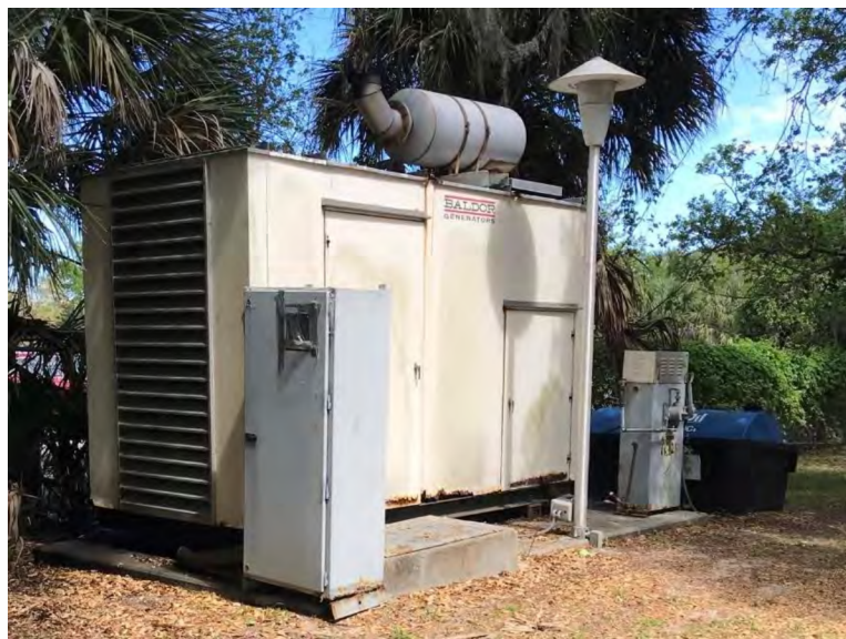
Figure 2-17: Emergency Generator
