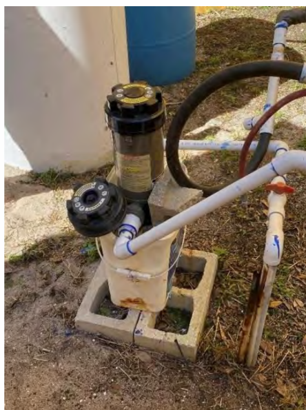
Figure 2-8: Hypochlorite Disinfection
