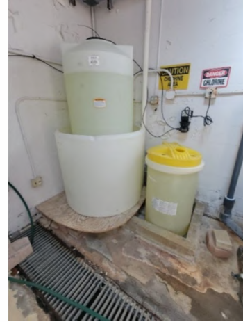
Before (Left) & After (Right): Chemical containment inadequate (note dry chemicals all over floor in before photo).
