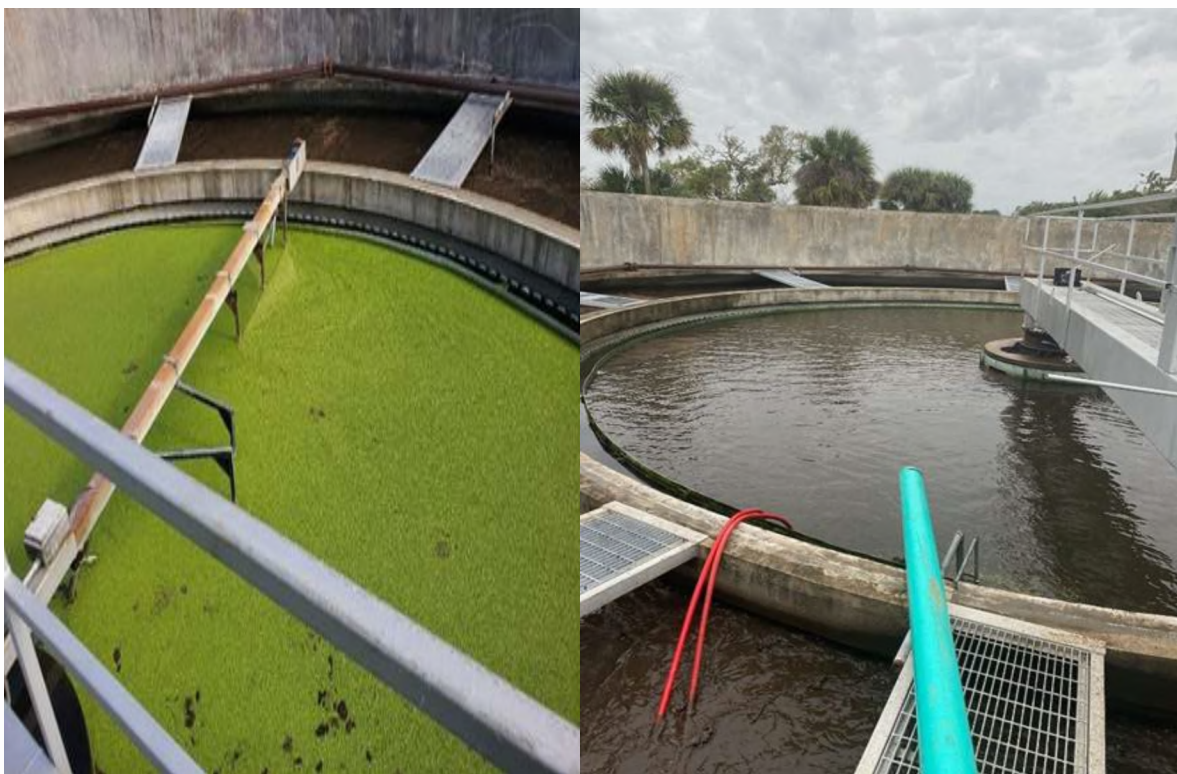
Before (Left) & After (Right): Skimmer repair fixing duckweed issues and improving clarifier performance.
