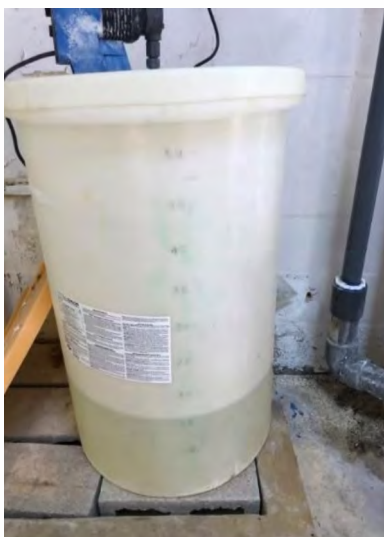
Figure 2-7: Chlorine Treatment
