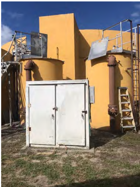
Figure 2-7: Sand Filters
