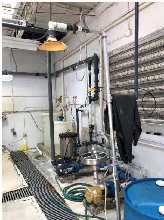
Figure 2-16: Emergency Shower, Drains, and Chemical Containment
