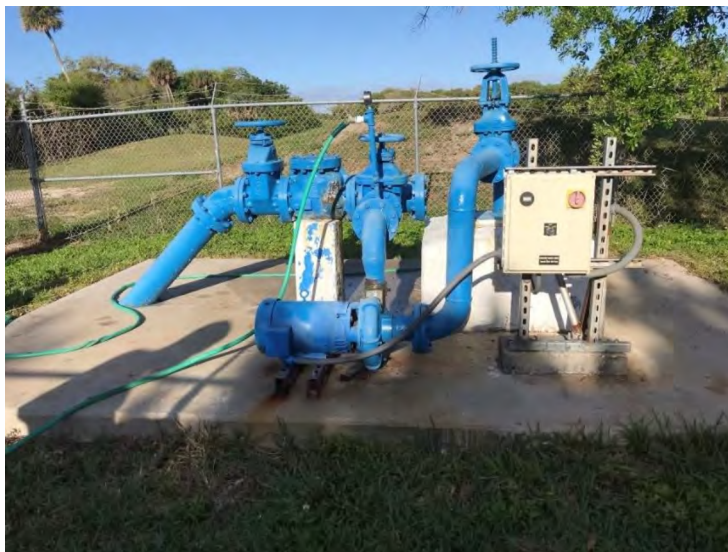
Figure 2-1: Well #1 Irrigation and Fire Suppression Well
