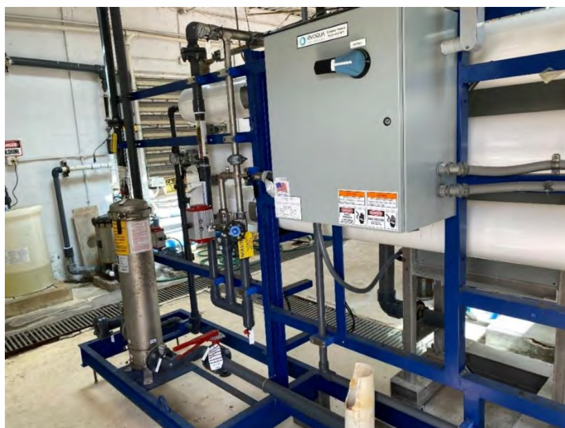
Figure 2-5: Vantage M83 RO System
