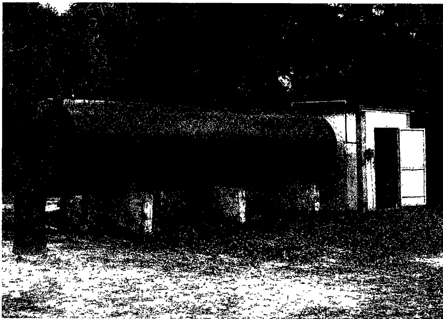
3,000-gallon Hydropneumatic Tank at at the Anclote Water System
