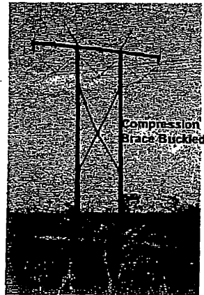
Figure 8 Structure #16Z59 Looking West
