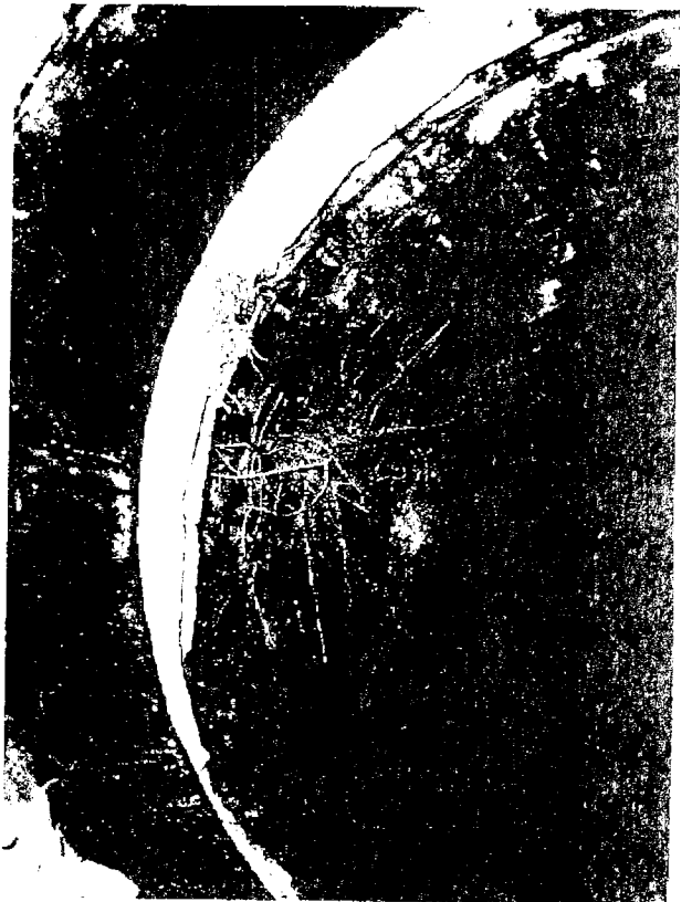
DEFECT: Roots through bricks need sealed & an inflow plug LOCATION: 2517
