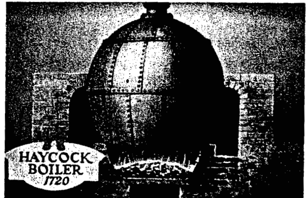
Fig. 5 The Haycock boiler
