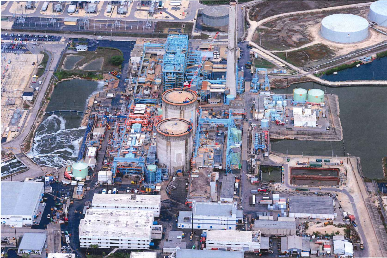
Aerial photograph of Turkey Point, Units 3 and 4. The photograph illustrates the extremely limited space in which to conduct these massive construction modifications.
