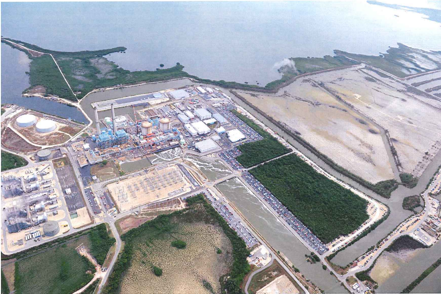
Turkey Point Unit 3 2012 outage site layout with thousands of workers on site. Note the close proximity of the fossil units 1 and 2 on the left to the nuclear units 3 and 4 and the close proximity of the water result in very little space for new plant components and pre-fabrication areas.
