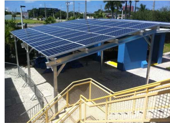
From second floor viewing area, PV house in background
