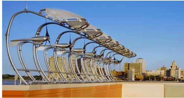
AVX1000 Building Integrated Wind Turbine (1 kW)
