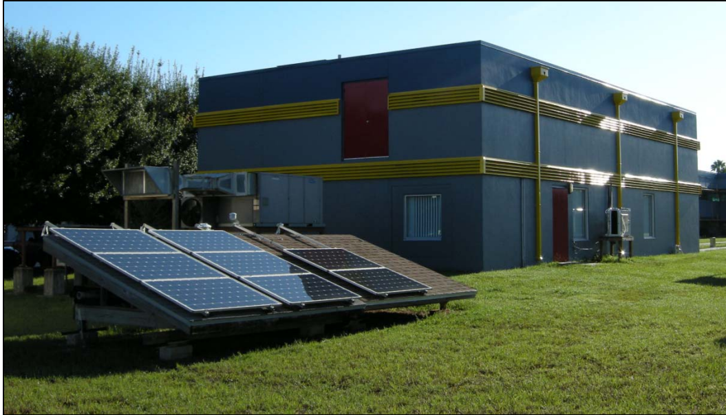
Figure 5. Building Science Lab building with 8 PV panels in the foreground. The outdoor unit of the 1.5-ton mini-split heat pump can be seen along the south wall of the building. Batteries, charge controller, inverter, and 8 batteries are located in a lab building room closest to the PV panels.
