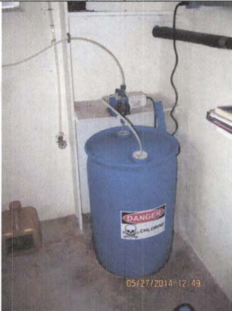
Chlorine Storage and Pump
