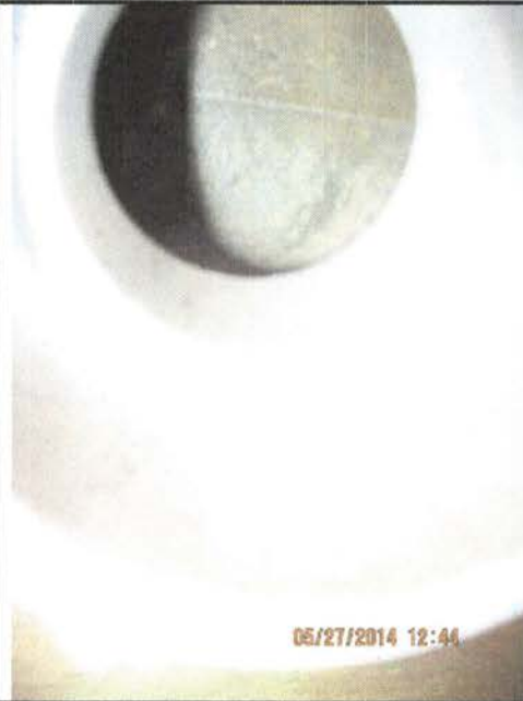
Well 1 (Eastern) – Pipe without mesh screen
