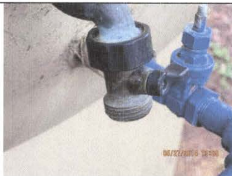
Treated Sample Tap on Hydro Tank
