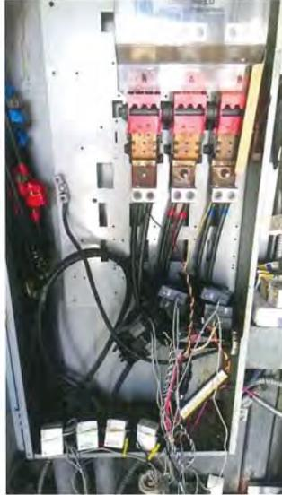
Figure 2 - Main Disconnect Panel
