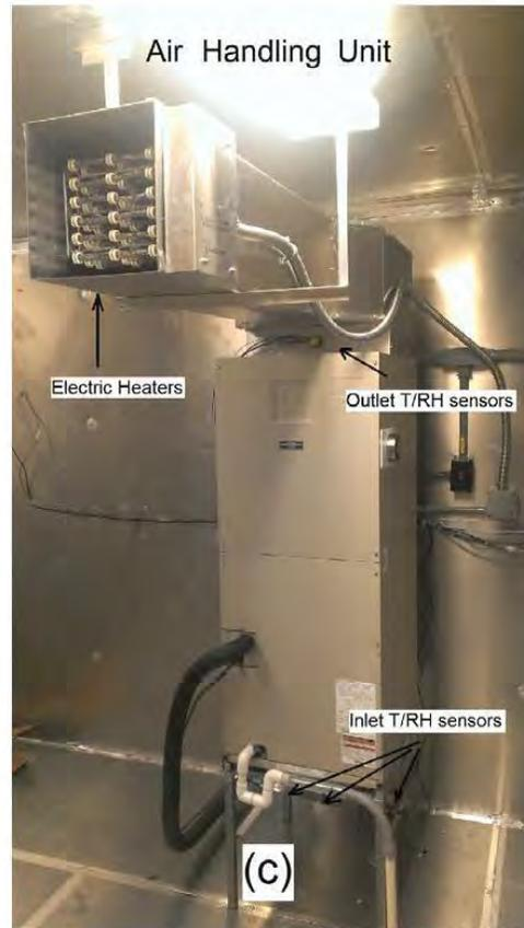
Figure 6: (a) solar collector, (b) condensing unit and (c) air handling unit
