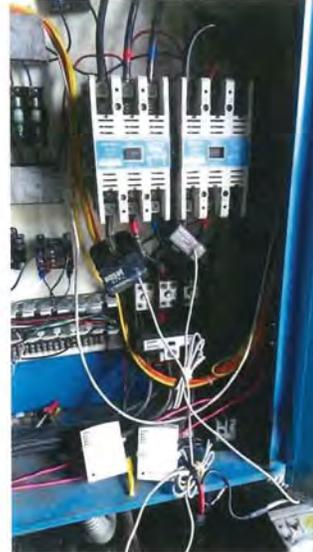
Figure 3 - Evaporator Fan Controllers
