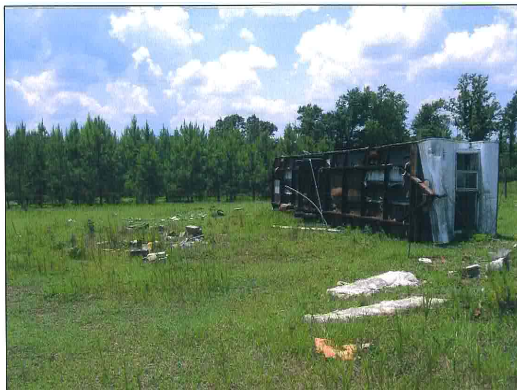
Photograph No. 30. View, looking southwest, of another demolished trailer located on the western portion of the subject property.
