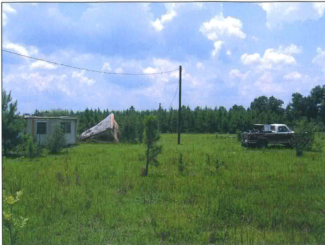
Photograph No. 29. View, looking south, of demolished trailers located on the western portion of the subject property.
