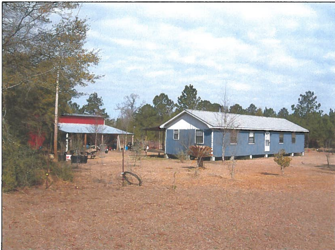
Photograph No. 6. View, looking northwest, of the residence and barn located on the south-central portion of the subject property.
