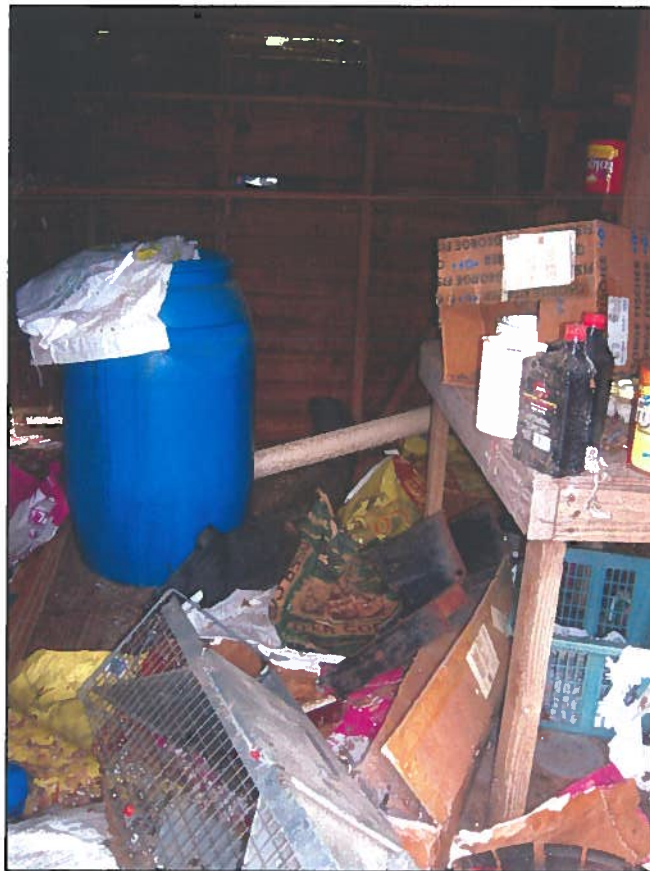
Photograph No. 36. View of the barn interior.
