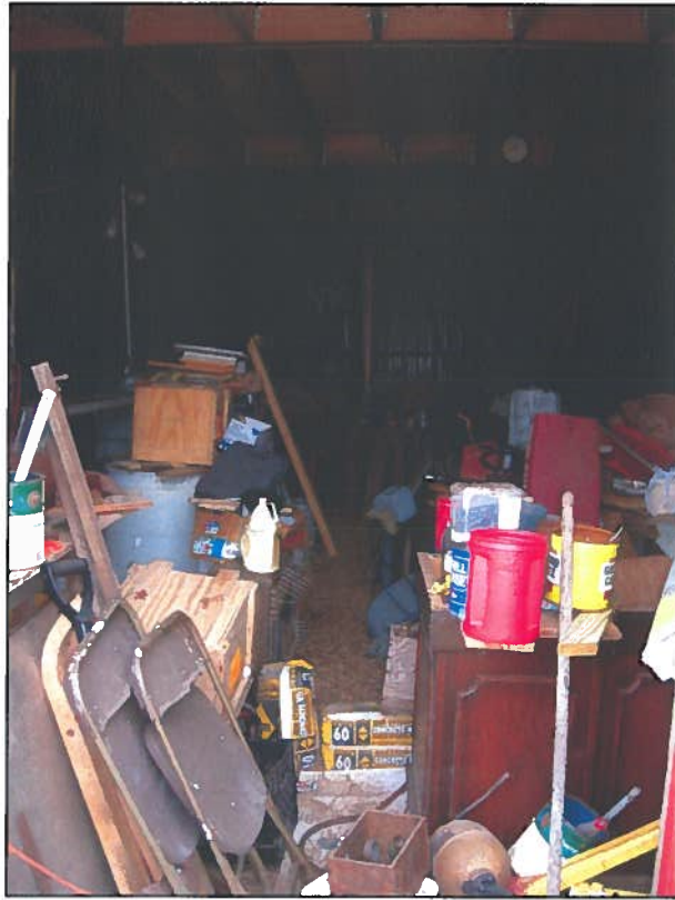
Photograph No. 35. View of the barn interior.
