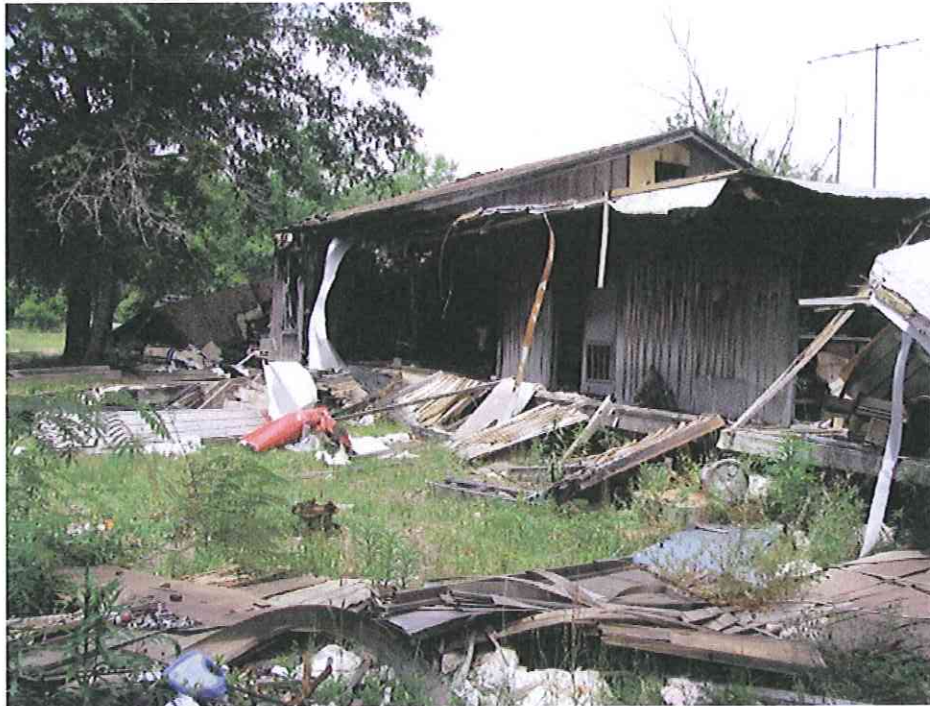
Photo Number 01: View of the Residence on the Comalander Parcel.
