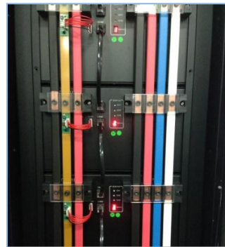
② Control power circuit breaker
