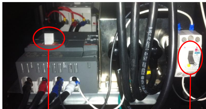
③ Main power circuit breaker
