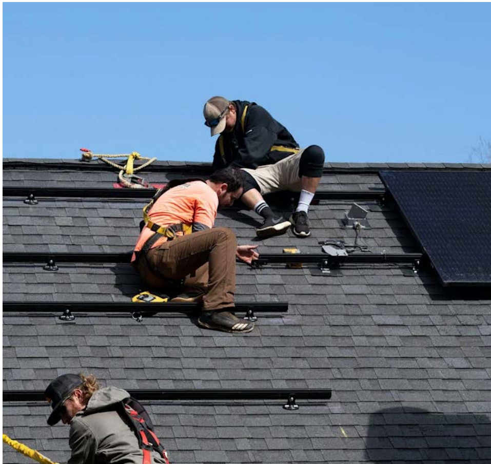
Sun Farm Energy workers on Feb. 8 install solar panels on a home in Escambia County.
