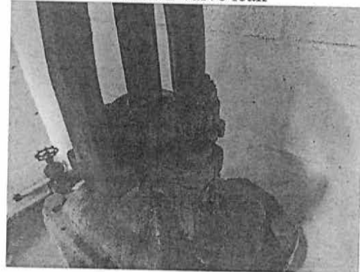
Well #2 valve leak
