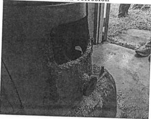
Well #3 corrosion
