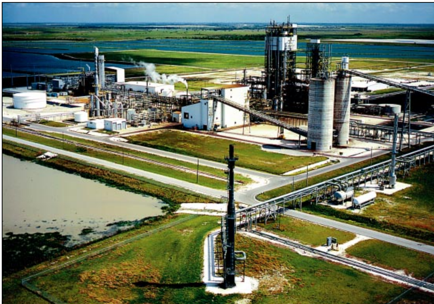
Aerial view of Polk Power Station
