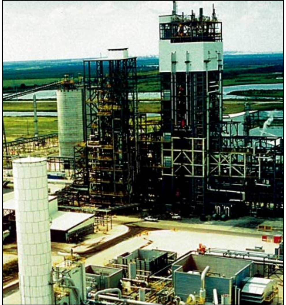
The Texaco gasifier is in the largest structure, which also contains the radiant syngas cooler. The hot gas cleanup system is installed in the smaller of the two large structures. In the foreground is the air separation unit.
