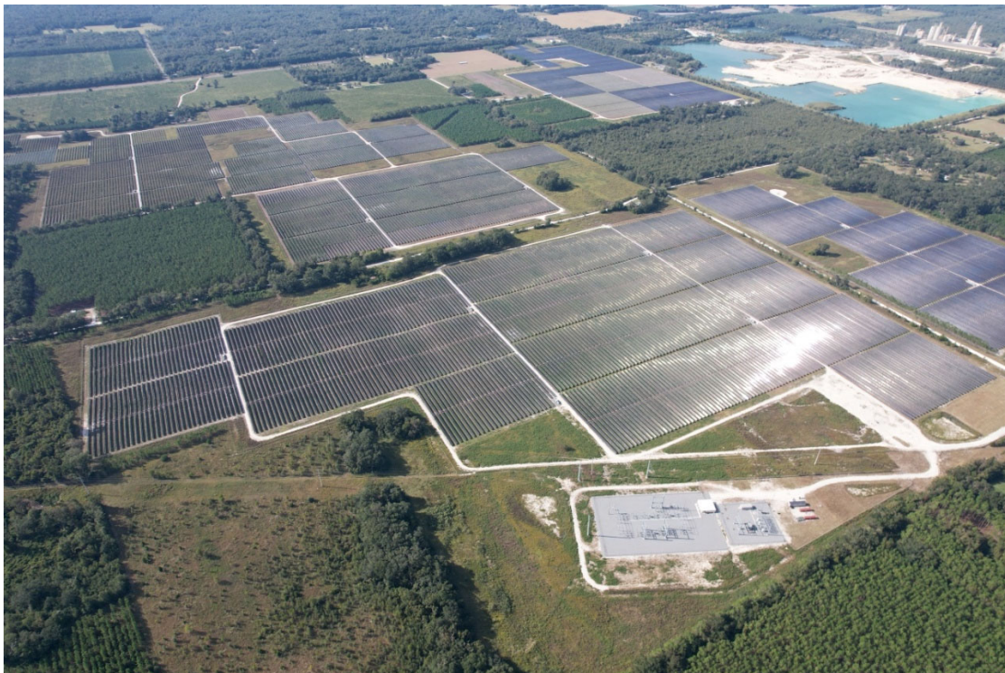
FIGURE 3.5 Hildreth Power Plant
