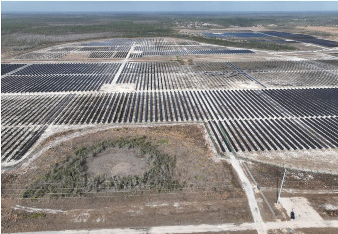
FIGURE 3.2 Bay Ranch Solar Power Plant
