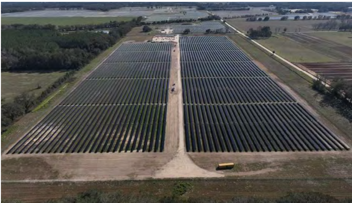
FIGURE 3.3 Hardeetown Solar Power Plant
