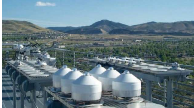
Figure 3-10. Kipp & Zonen model CM22 pyranometers installed in ventilated CV2 enclosures. Photo by NREL
