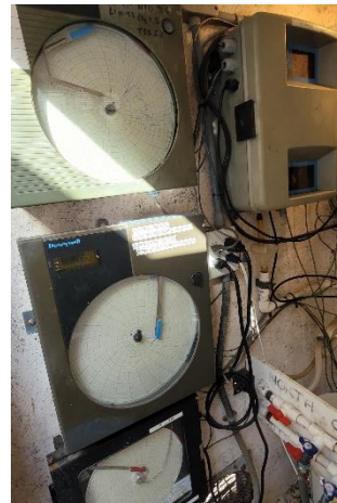
Chart recorders: flow, turbidity, and chlorine
