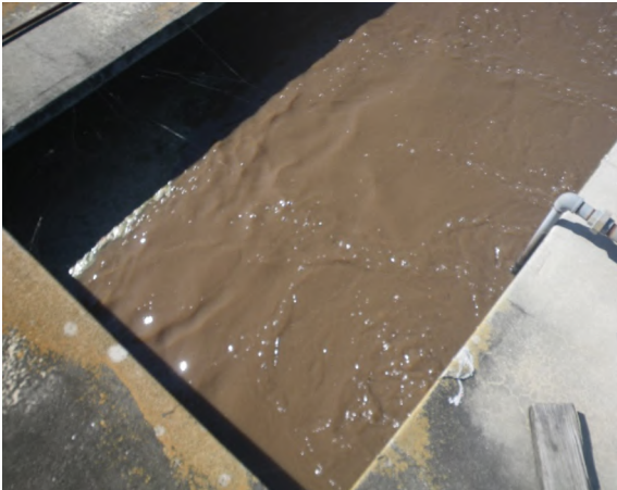
9 Dead spot at diffuser in third basin
