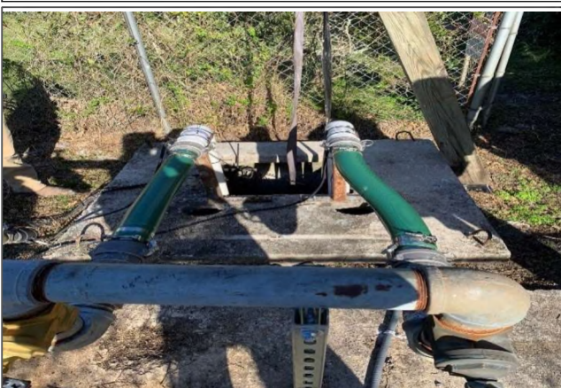
36. Lift station temporary pumps
