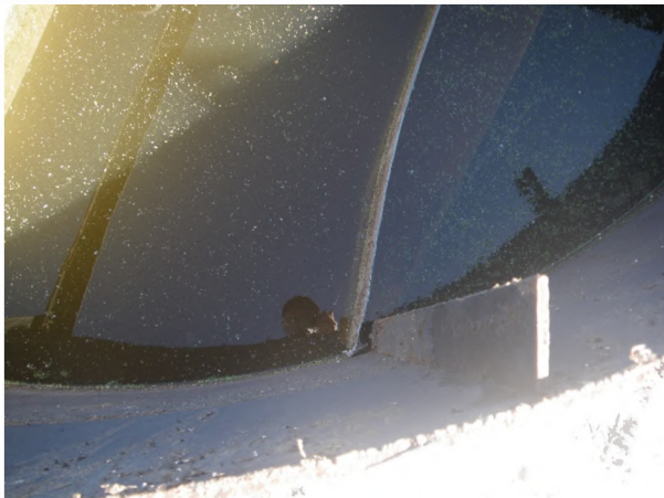
15 Separated baffle in CCC
