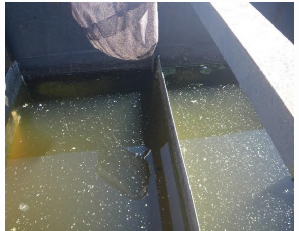
16 Separated baffle in CCC
