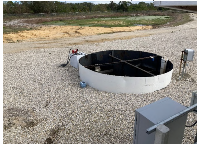
24. Chlorine Contact Chamber (CCC)
