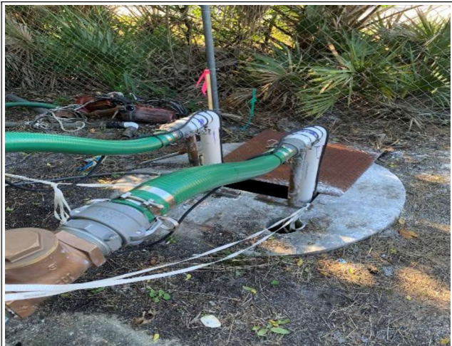
32. Lift station temporary pumps
