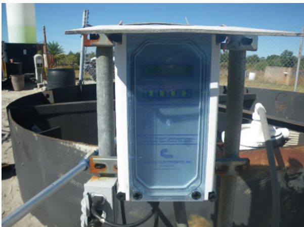
17 Ultrasonic flow meter
