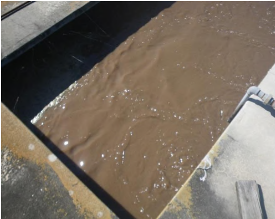
9 Dead spot at diffuser in third basin
