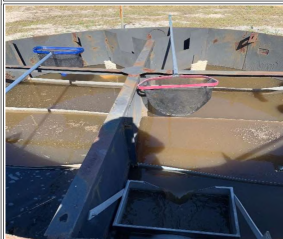
23. Chlorine Contact Chamber
