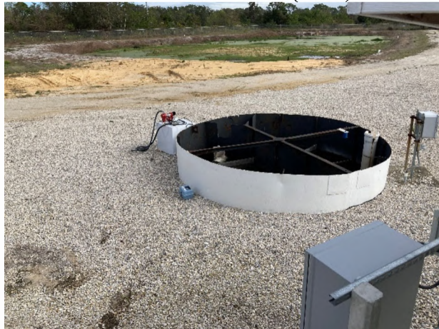
24. Chlorine Contact Chamber (CCC)
