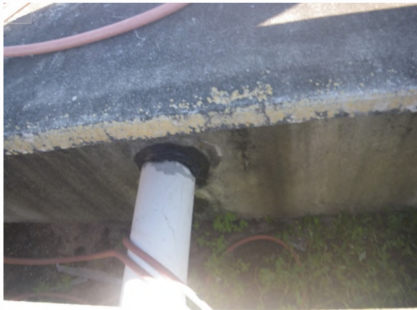
12 Leak around pipe connection
