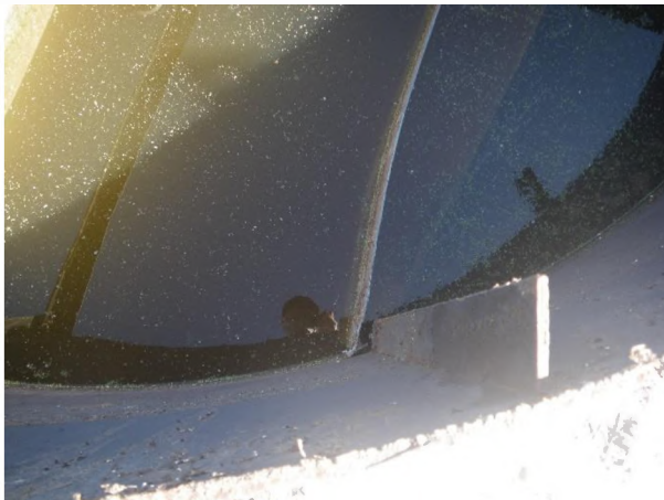
15 Separated baffle in CCC
