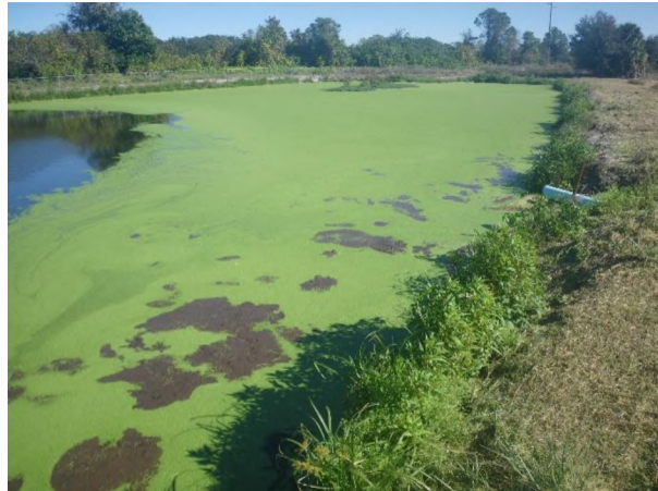
2 Sludge in percolation pond
