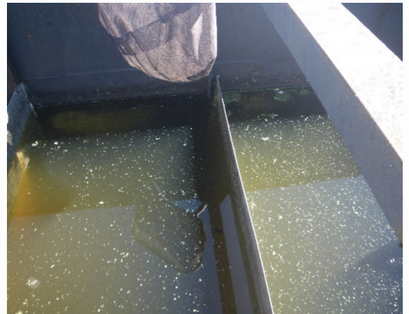
16 Separated baffle in CCC
