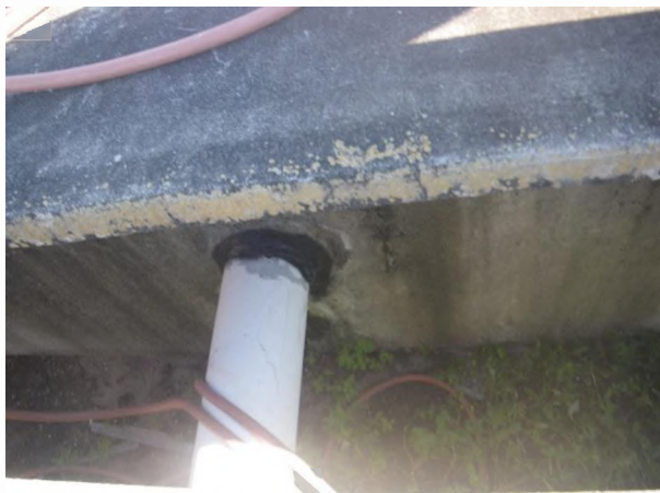
12 Leak around pipe connection
