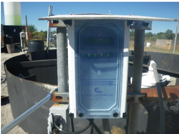
17 Ultrasonic flow meter
