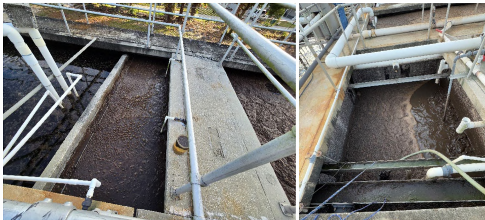
13 14 PVC aeration piping throughout facility to be replaced with proper materials.
