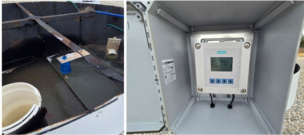
New ultrasonic flow meter in weir box (left) and meter controller (right).
