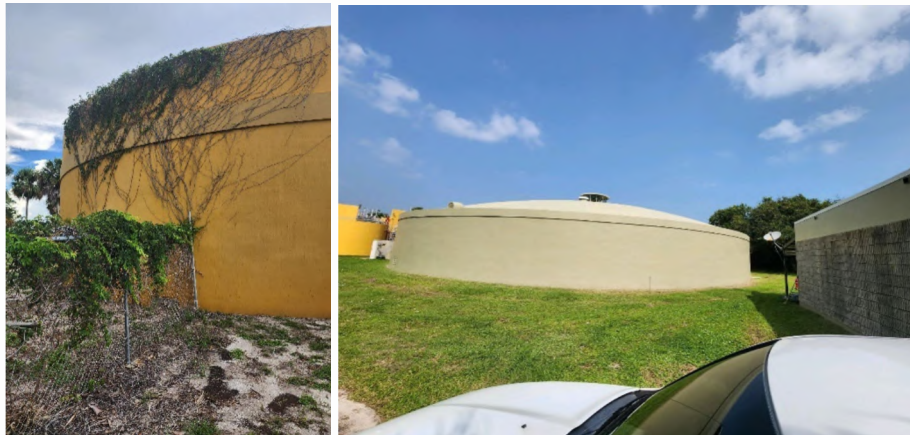
11 12 Irrigation and Fire Control Ground Storage tank before (left) and after (right) before and 13 after inspection and recoating, note vegetation overgrowth removed from tank.
