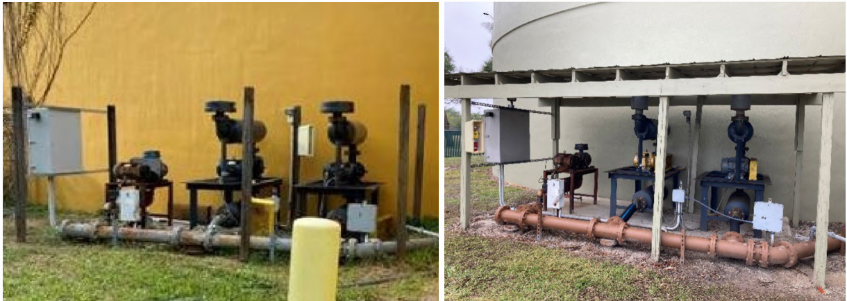
7 8 New Shade structure over Aquarina blowers before (left) and after(right) improvement.
