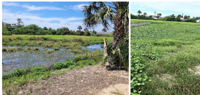
Examples of overgrowth of vegetation in rapid infiltration basins.
