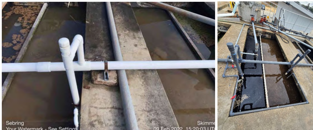
14 Old skimmer and air lifts (left) and newly installed air lifts and sludge returns (right), note
