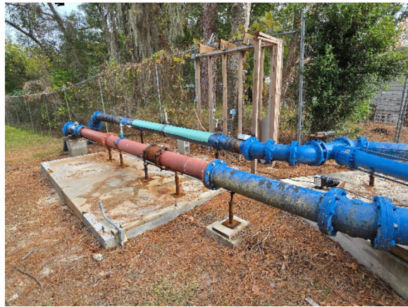
Replaced segment of above ground piping
