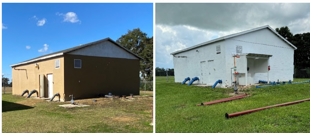
7 8 Treatment, pumping, and control building before (left) and after (right) recoating.
