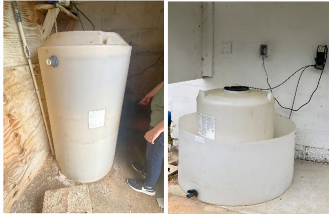
4 5 Chlorine storage before (left) and after (right) installation of spill containment.
