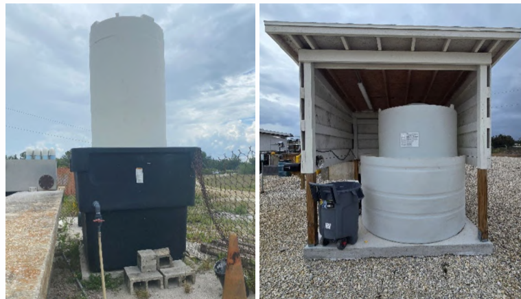
14 15 Disinfection chemical storage before (left) and after (right) improvement.
