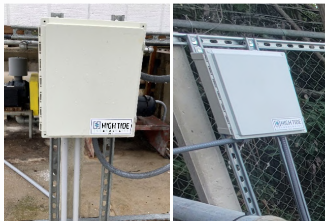
Remote monitoring equipment installed at the wastewater treatment plant (left) and lift stations (right).
