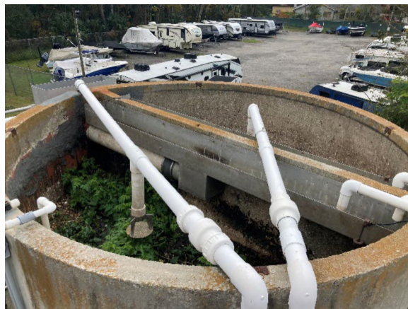
Sand filter with impacted sludge allowing vegetation growth.
