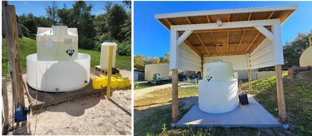
5 6 Chemical storage before (left) and after (right) improvement.
