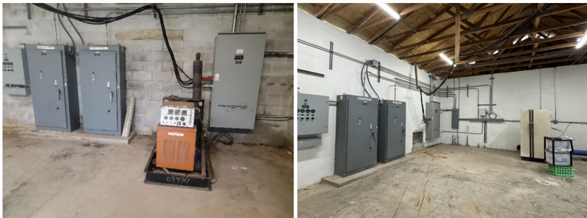
Before (left) and after (right) removal of stationary generator. Also note painting of building interior.
