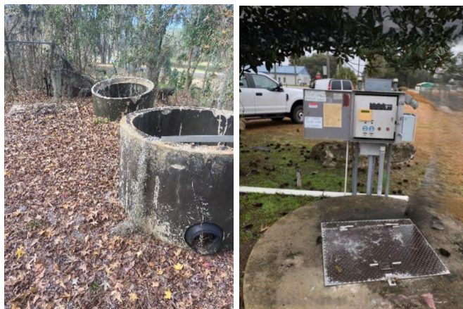
11 12 Damaged unused manhole rings, trash, and vegetation overgrowth at Tradewinds lift station 13 site, including vegetation causing fence damage (left). Tradewinds lift station lacking 14 fencing (right).
