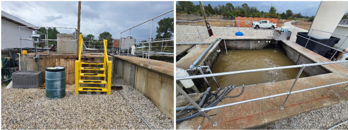
New access stairs with handrails, high friction tread plates, high visibility coating (left) and new fall protection rails around the exterior of the facility to prevent falls from the plant (right).
