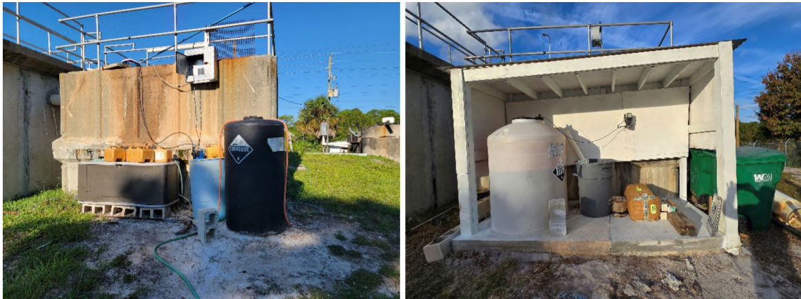
7 8 Chemical storage before (left) and after (right) improvement. Note dead grass and chemical 9 storage around old tank indicating chemical spills and disorganized arrangement.
