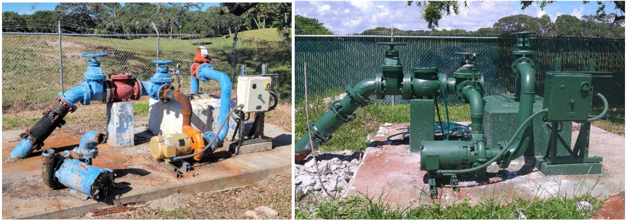
Example of before (left) and after (right) repainting of above ground piping and equipment.
