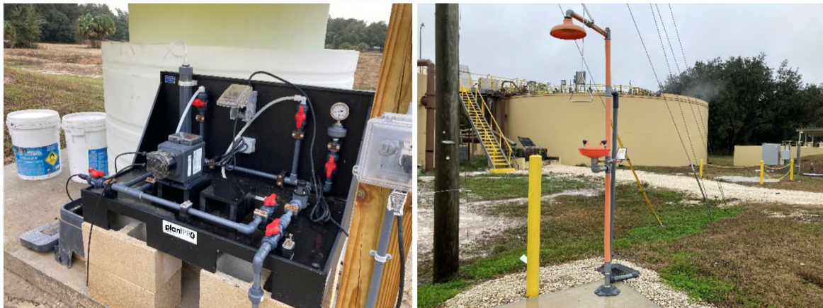
7 8 New variable chemical dosing pump (left) and emergency chemical shower and eyewash 9 station (right)
