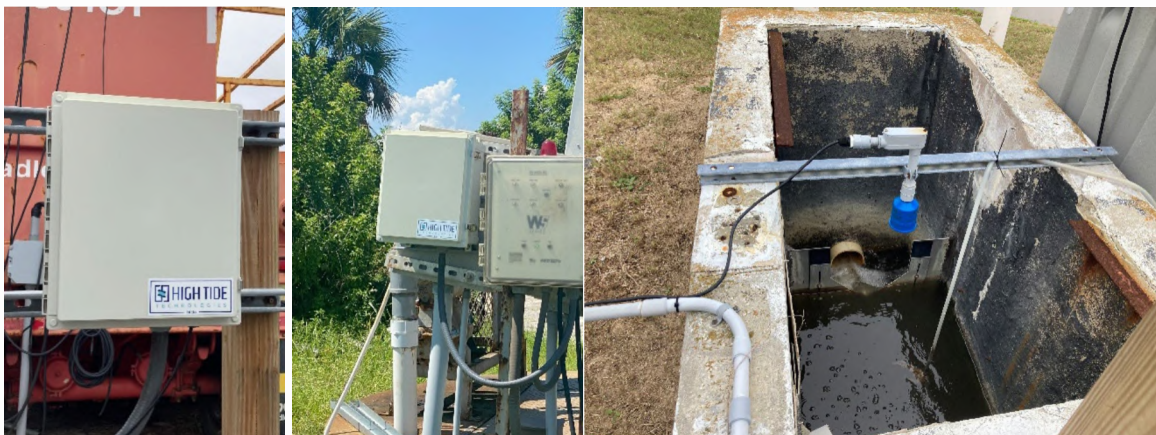
New remote monitoring units installed at the treatment plant (left) and lift stations (center).
