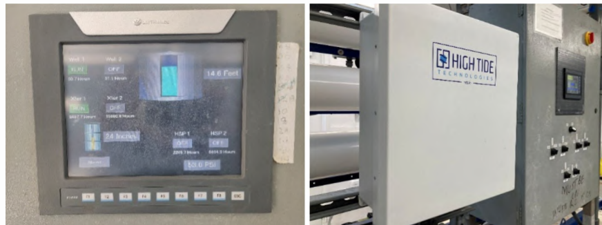
Telemetry with tank levels (left) and new remote monitoring equipment (right).
