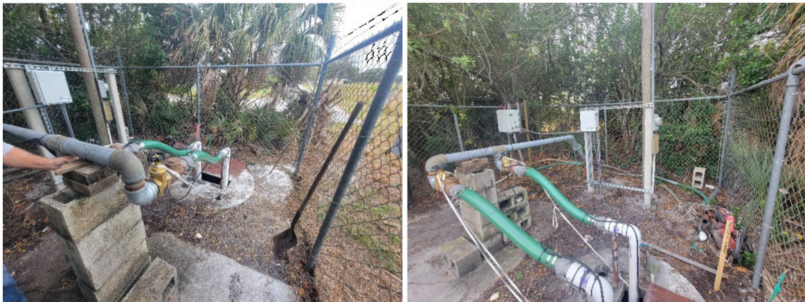
Example of lift station piping and condition currently.
