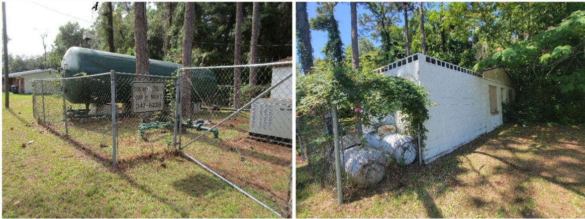
1 2 Sun Ray Estates (FL3421314) well and hydro-pneumatic storage tank (left). Generator and 3 disinfestation shed (right).
