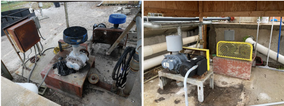
8 Blowers before (left) and after (right) improvements.
