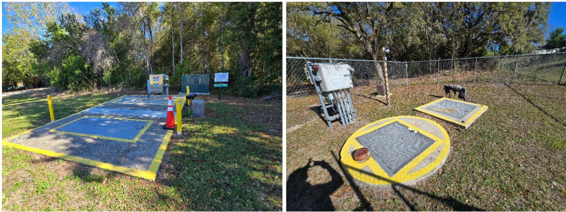
Examples of high visibility paint application to tripping hazards.
