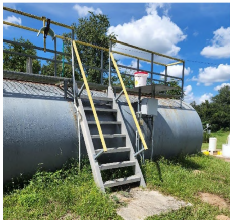
Disinfection mixing tank before (left) and after (right) recoating and repainting handrails
