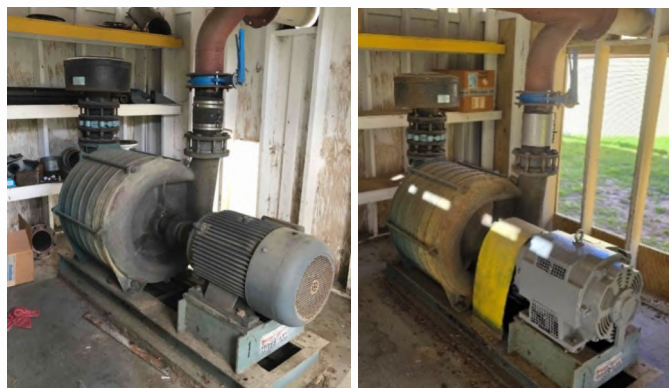
13 14 Blower motor before (left) and after (right) replacement, also repair work to blower building 15 underway at time of photo.
