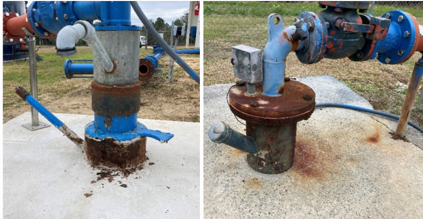
Well 2 (left) and well 3 (right) showing rusting on well columns, damaged coatings on attached equipment, exposed wiring, etc.
