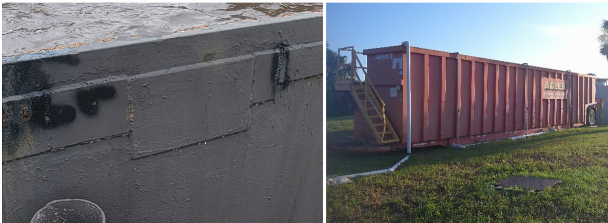
14 15 Example of patching leaks in steel tanks at North Peninsula (left) Temporary tank in place 16 since concrete tank failure (right).
