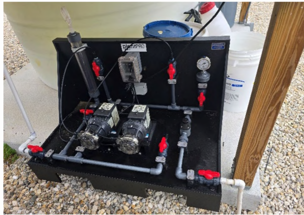
New chemical feed pump system for precise dosing of sodium hypochlorite.
