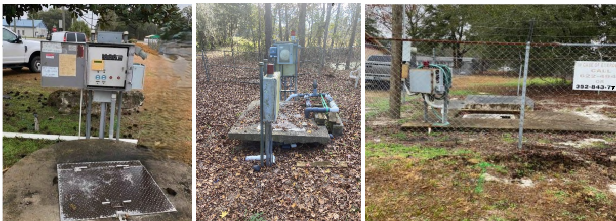
Examples of older Tradewinds collection system lift stations. Some lift stations lacked fencing, remote monitoring, and had rusting or degraded assets.
