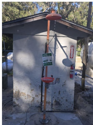
Emergency eye wash and chemical shower station and fires extinguisher - Ashley Heights
