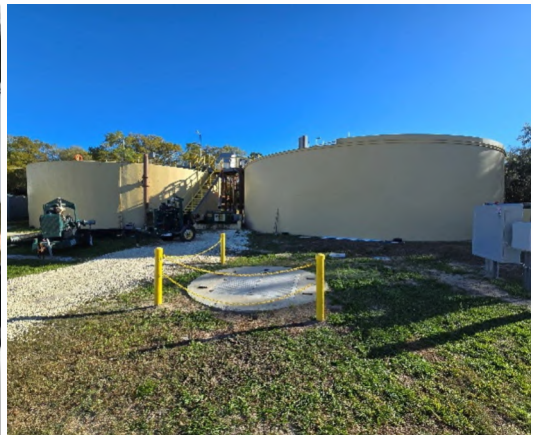
Facility tanks before (left) and after (right) recoating.
