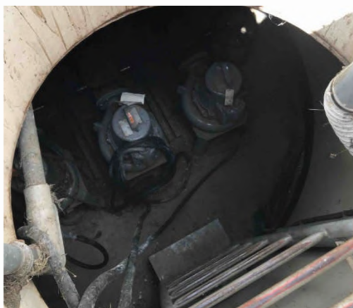
Lift station 2 dry well basin
