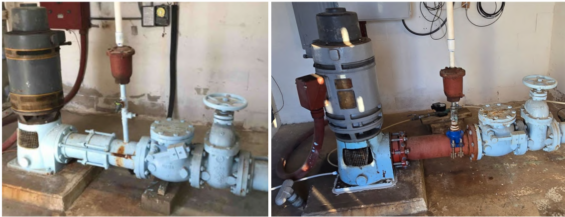
1 2 Well 6 before (left) and after (right) rehab work. Motor and pump serviced, leaking section 3 cf pipe replaced.
