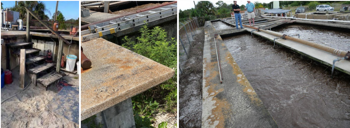
Examples of inadequate safety features for operations access. Rotting wooden stairs with missing handrail on one side (left), aluminum ladder resting across tanks for access to air header (center), no leading edge protection or grating over open basins throughout plant (right).
