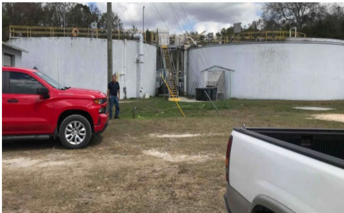
Facility tanks before (left) and after (right) recoating.
