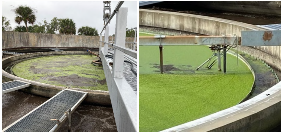
Examples of accumulation of duckweed growth in clarifier (left and right) including duckweed passing over the trough (right).
