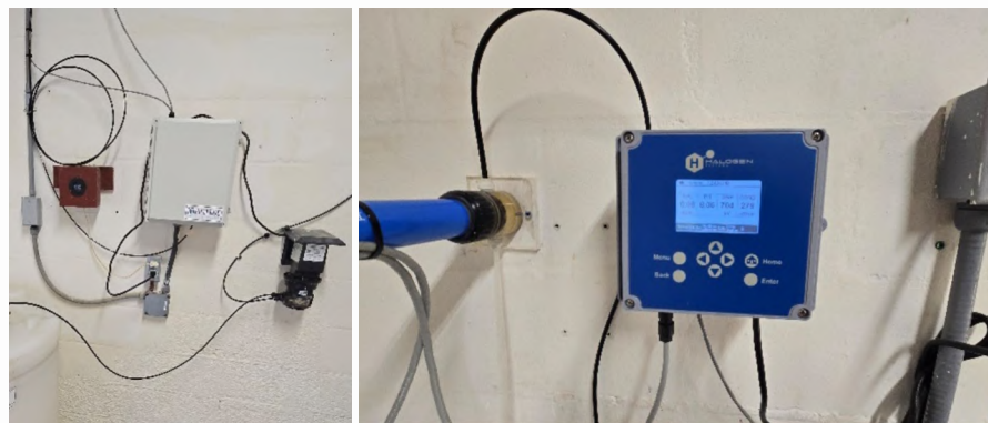
Examples of remote monitoring unit installed at each well site (left) and new chlorine residual monitoring equipment installed at each well site (right) (examples from Well 8 site).
