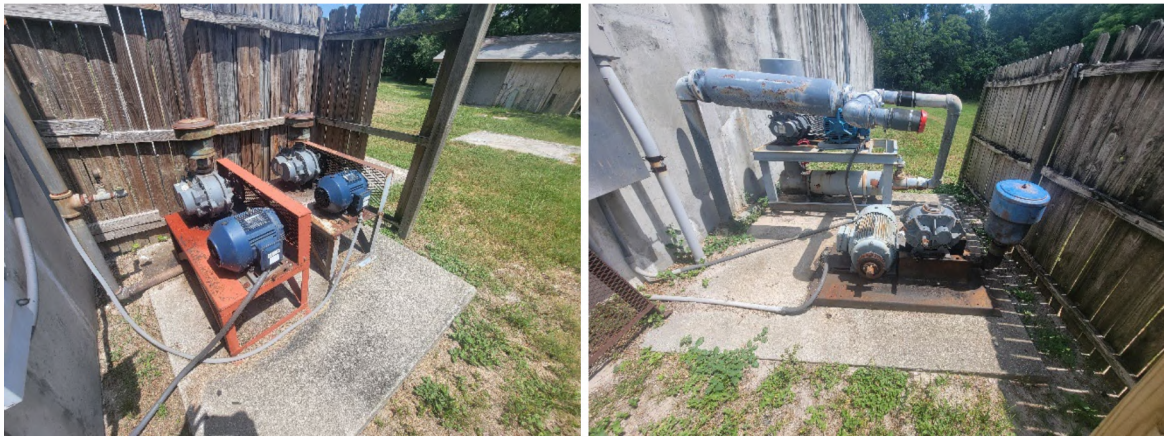
Surge basin / digester blowers (left) and aeration basin blowers (right)
