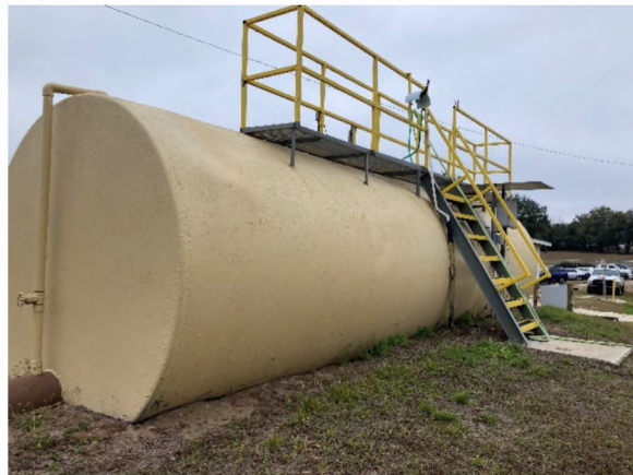
Disinfection mixing tank before (left) and after (right) recoating and repainting handrails
