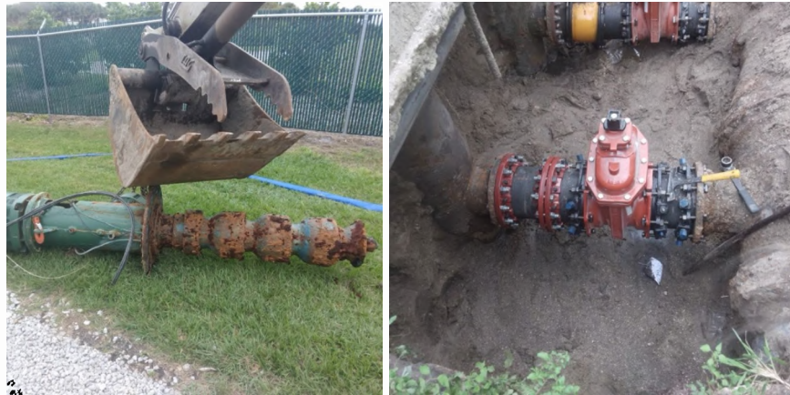
5 6 Rusted high pressure fire protection valves (left) removed and new valves installed (right)
