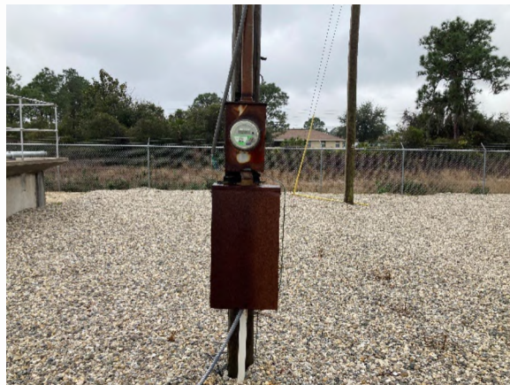
Extremely corroded existing 200 amp power supply.
