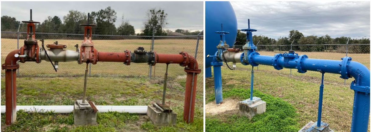
3 4 Hydro-pneumatic tank before (left) and after (right) recoating.
