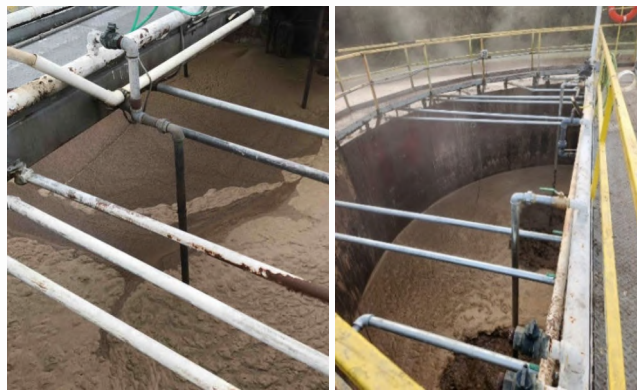
11 12 Examples of Aeration headers and drop pipes before and after replacement.
