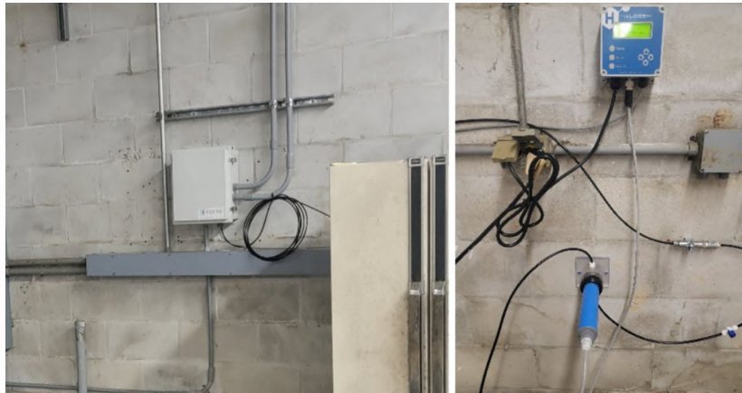
New Remote monitoring unit (left) and continuous chlorine analyzer (right).
