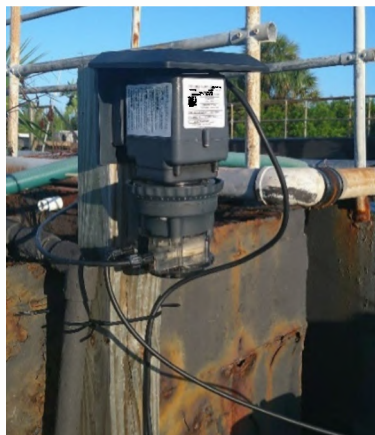
9 10 Repaired chemical feed pump.
