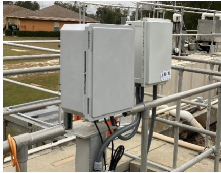
5 6 Newly installed remote monitoring equipment at the Landfair facility and lift stations 7 (example at treatment plant)
