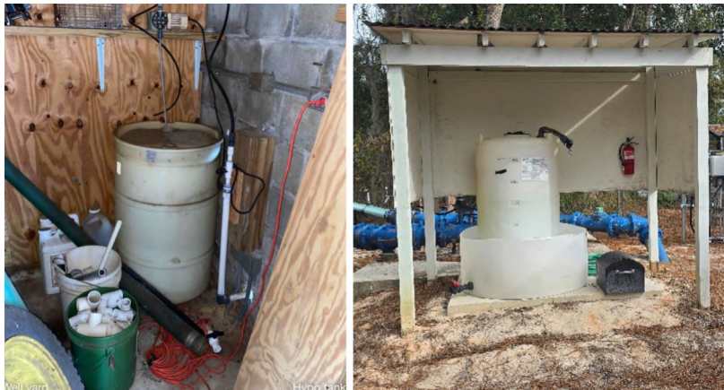
12 13 Disinfection system before (left) and after (right) improvement.
