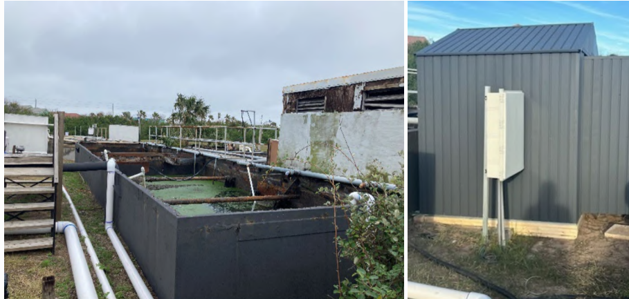
4 5 New temporary PVC aeration and sludge return lines throughout facility (left). Sound 6 dampening shed installed around blowers (right).
