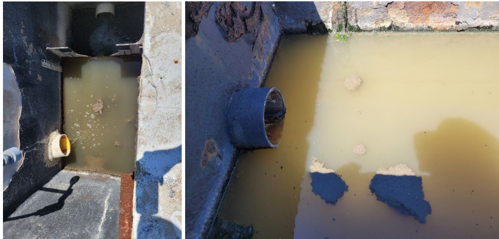
Discolored effluent and floating sludge at discharge at acquisition, indicating poor treatment.
