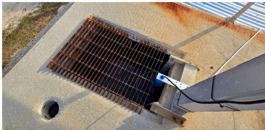
Covers replaced or added to ensure operator safety.
