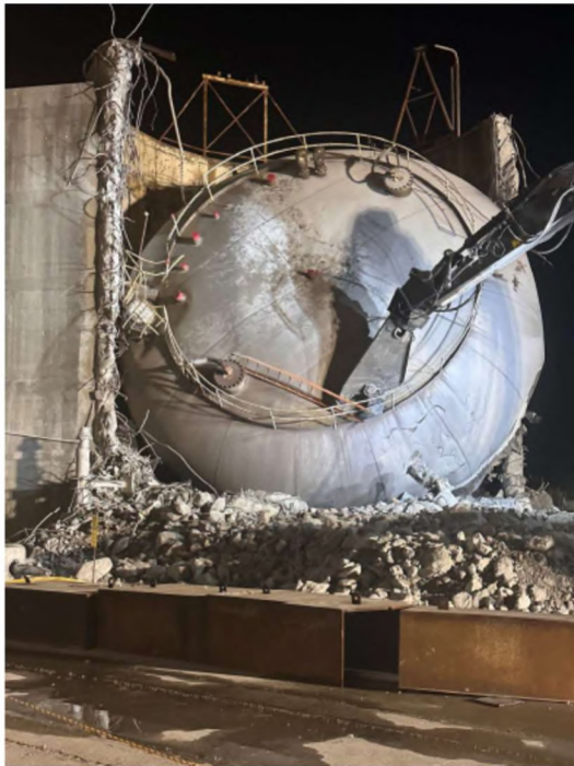
BWST- Steel Tank Demolition
