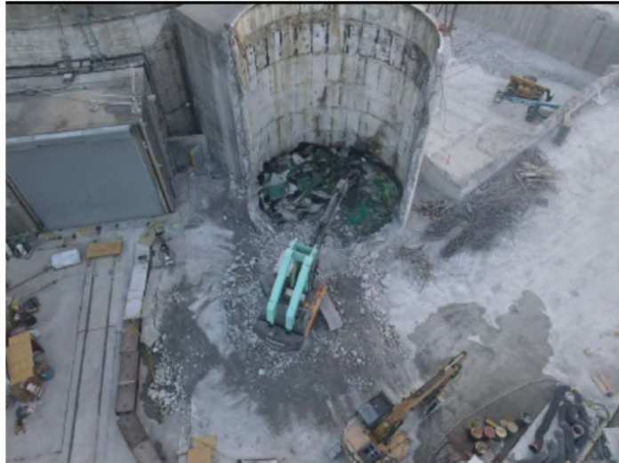
BWST Concrete Shell demolition
