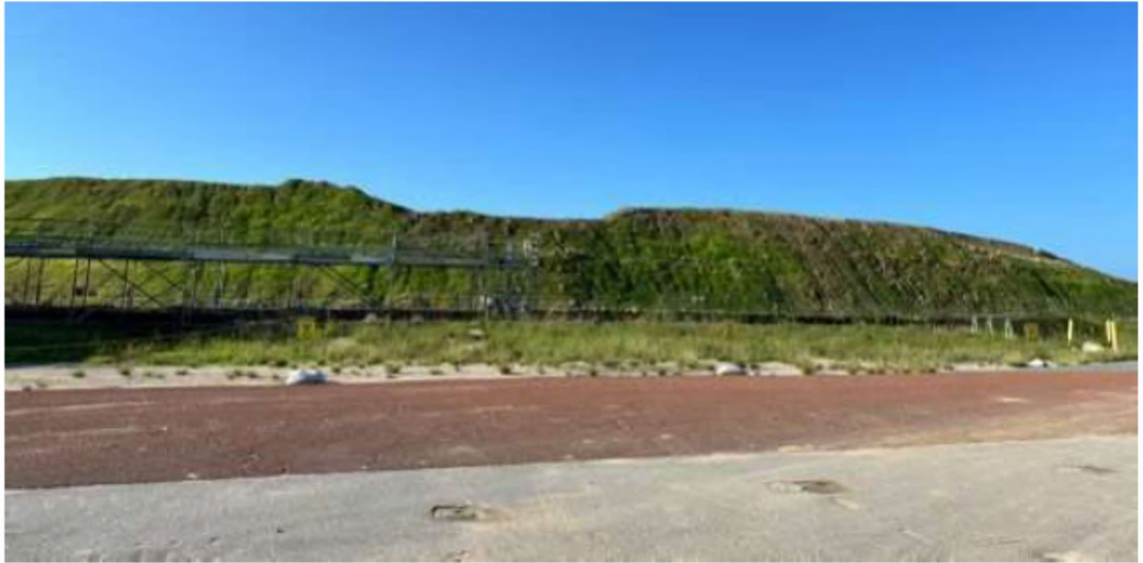
Stockpile Backfill Area 1
