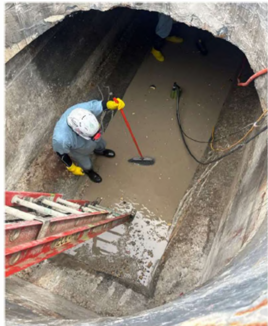
Cleaning out the Intakes
