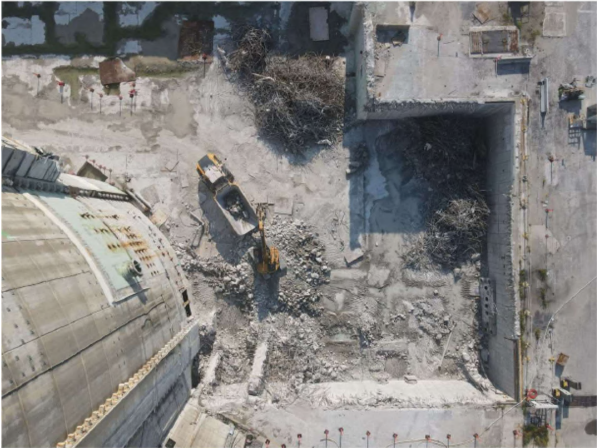
Seawater Room Demo Complete Steel & Concrete Loadout
