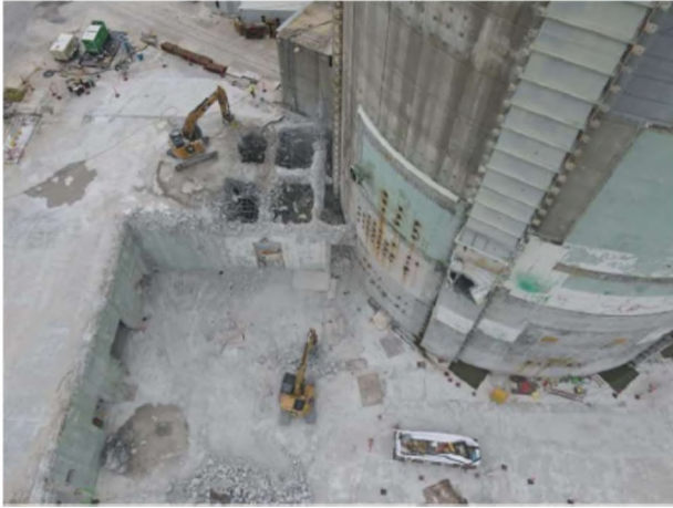
Seawater Room Roof Demo
