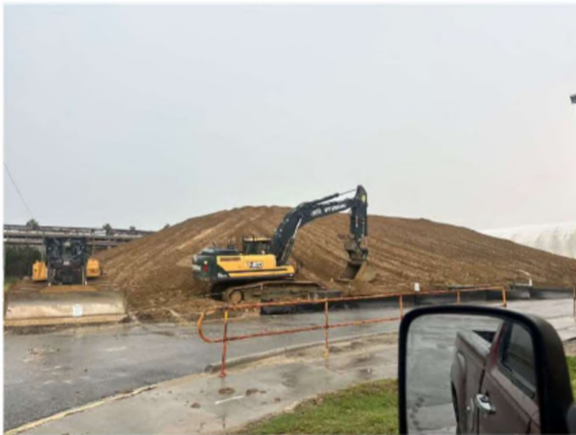
Stockpile Backfill Area 2
