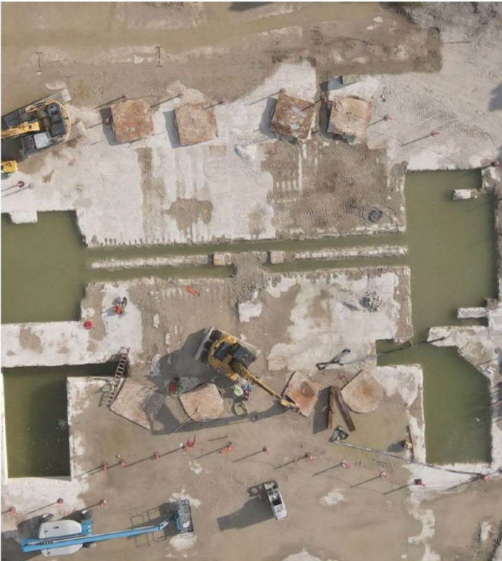
TB Circ Water Intake and Discharge Cleanout
