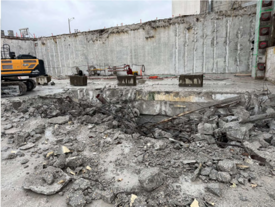
Decay Heat Vault Roof Demo
