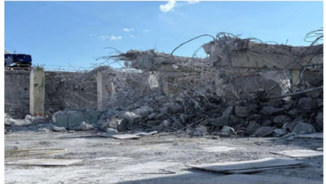
Seawater Room Wall Demo
