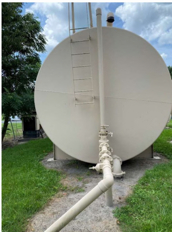
Figure 2-6: Ground Storage Tank 1
