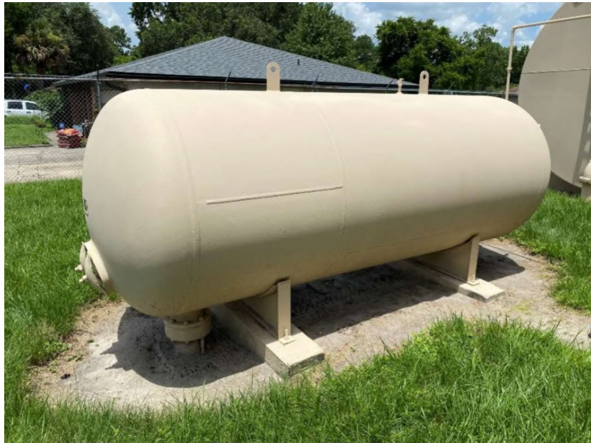
Figure 2-7: Hydropneumatic Tank
