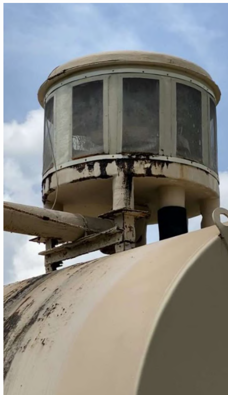
Figure 2-4: Aerator Treatment
