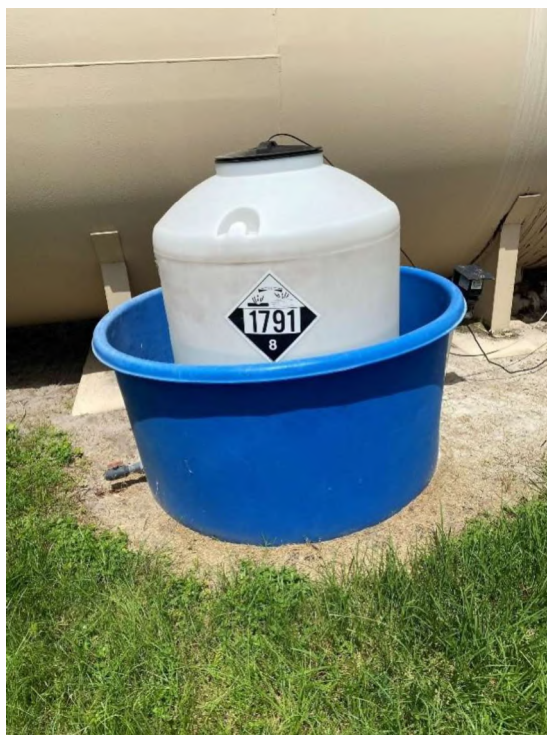
Figure 2-3: Sodium Hypochlorite Treatment
