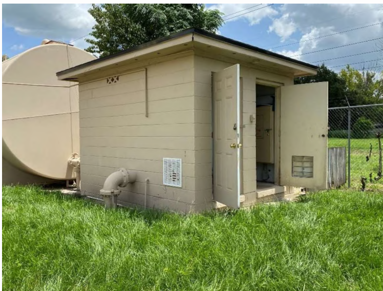
Figure 2-10: Pump Station Building
