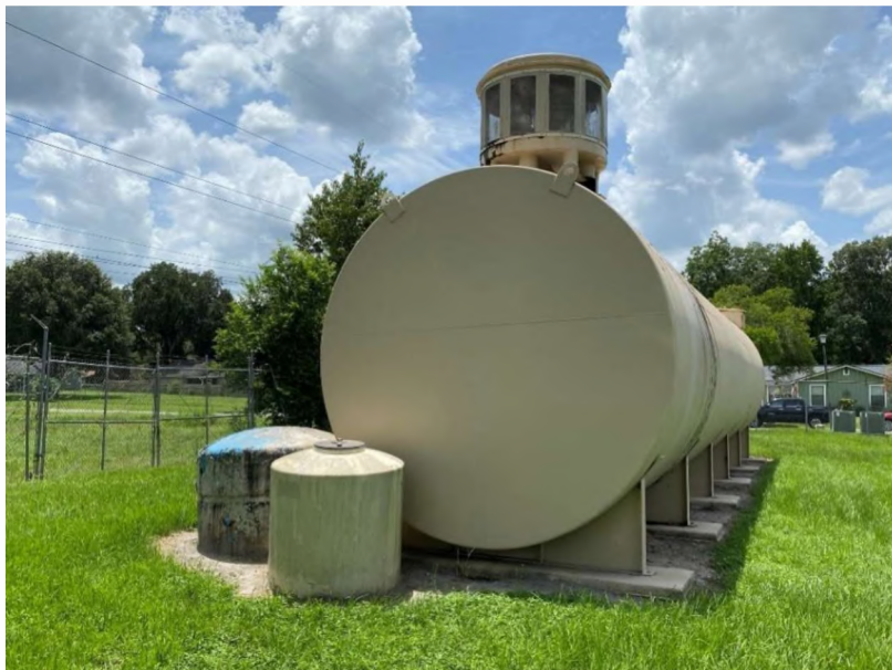
Figure 2-5: Ground Storage Tank 2
