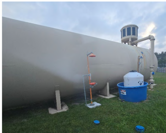
Exterior recoating completed on Tank 2 and the aeration unit.
