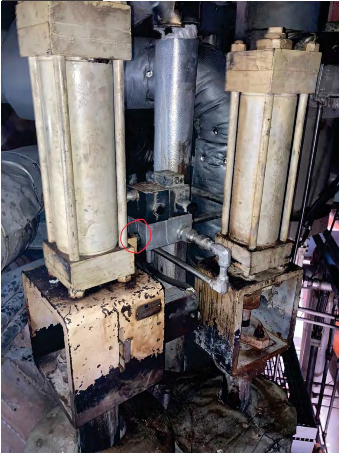
Figure 1 BPFDV and VV valves with fittings
