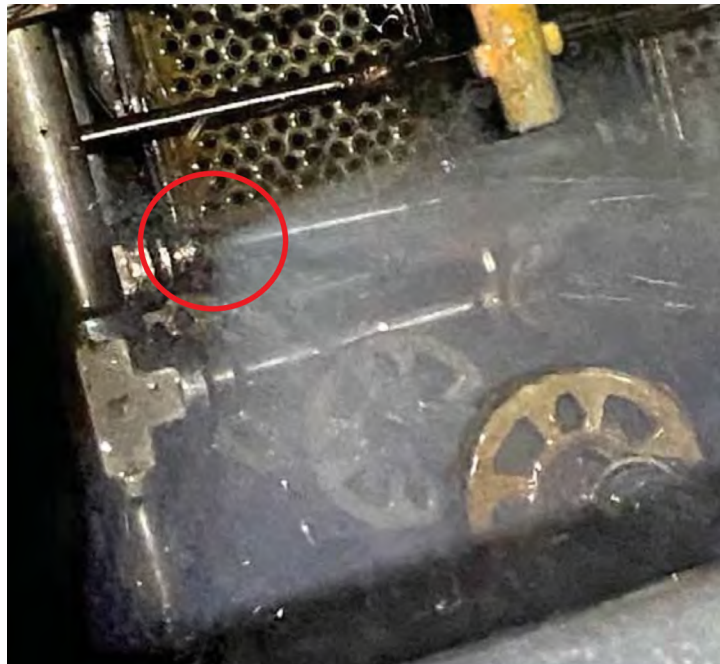
Figure 1 Failed weld on BPFDV line
