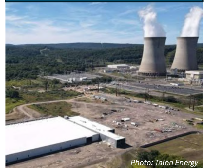
Susquehanna Nuclear Plant and Data Center
