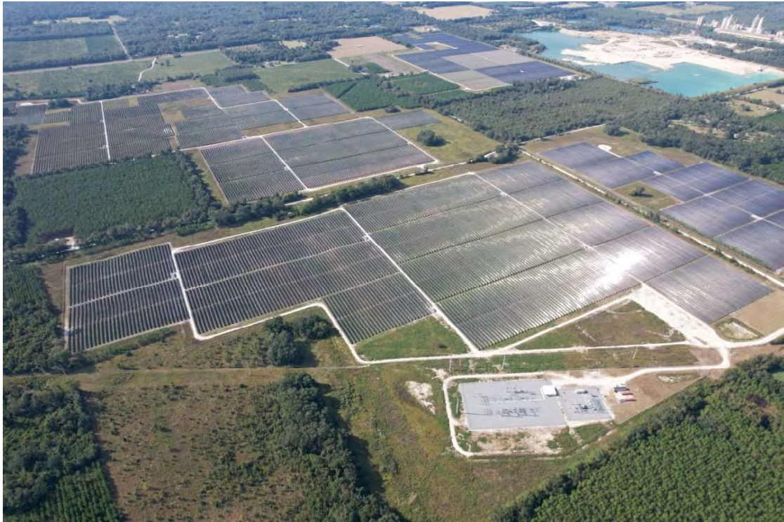
FIGURE 3.5 Hildreth Power Plant
