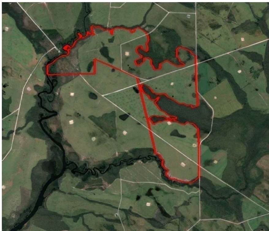
FIGURE 4.1 Mule Creek Solar Project
