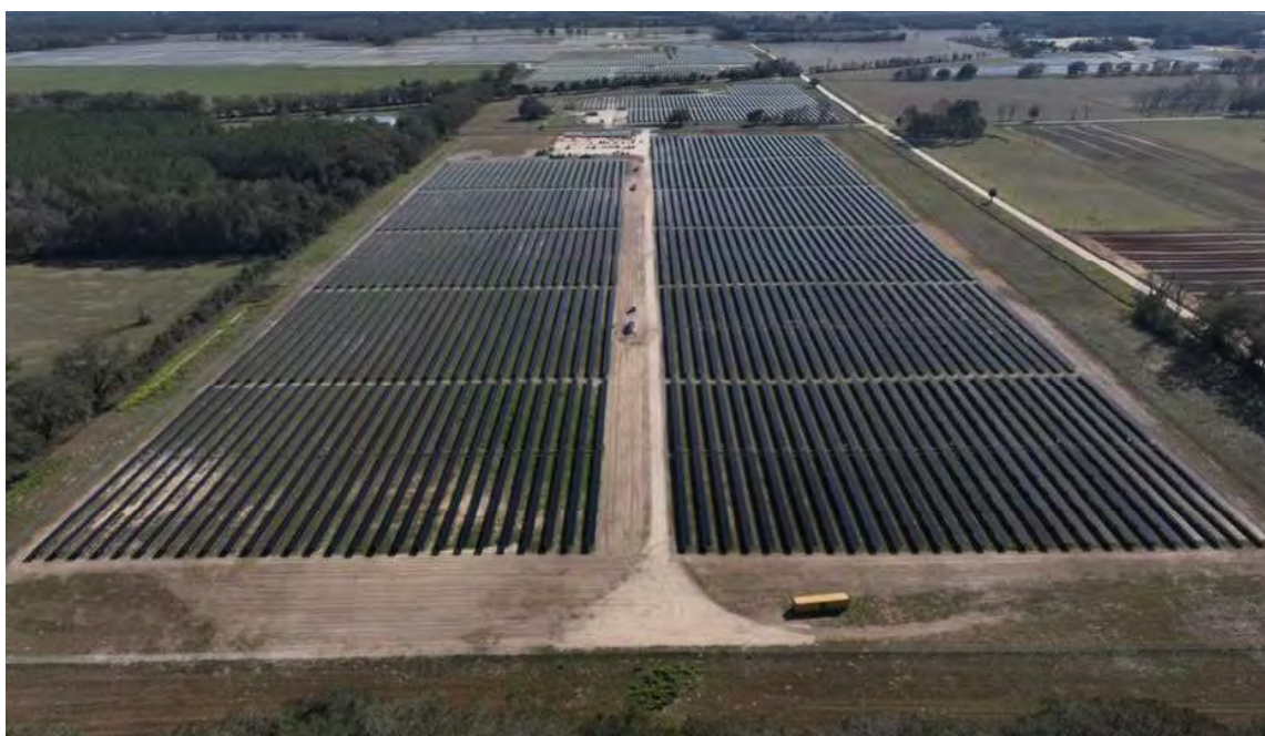
FIGURE 3.3 Hardeetown Solar Power Plant
