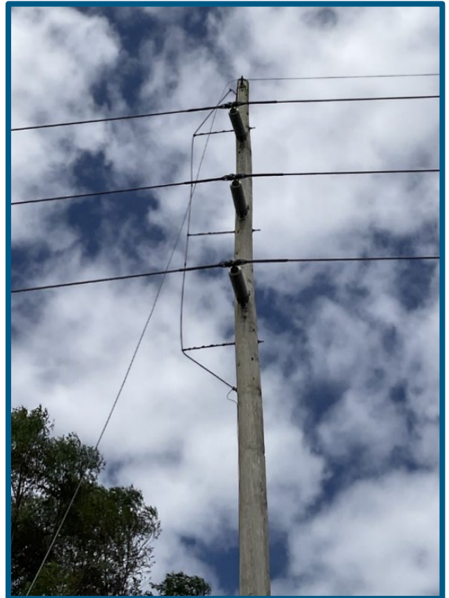
Figure 2: Broken Static due to extreme weather event.
