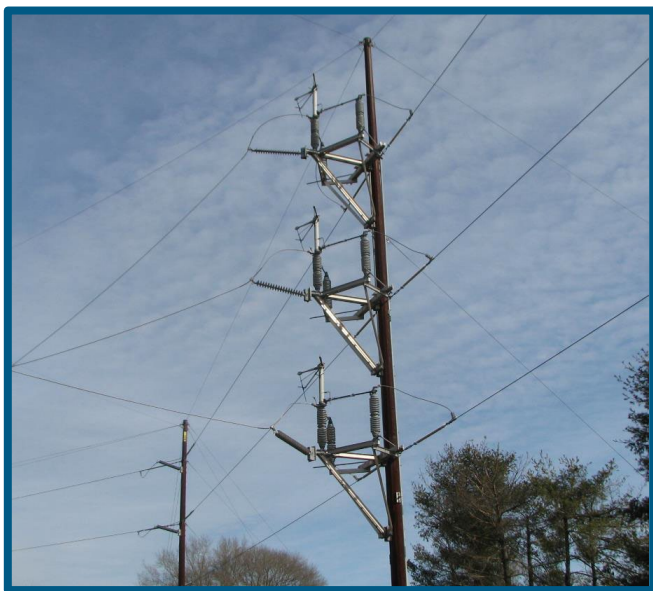
Figure 5: DEF Manually Operated Switch
