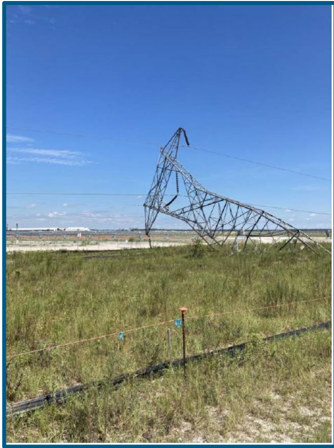
Figure 4: Lattice Tower impacted by Hurricane Idalia
