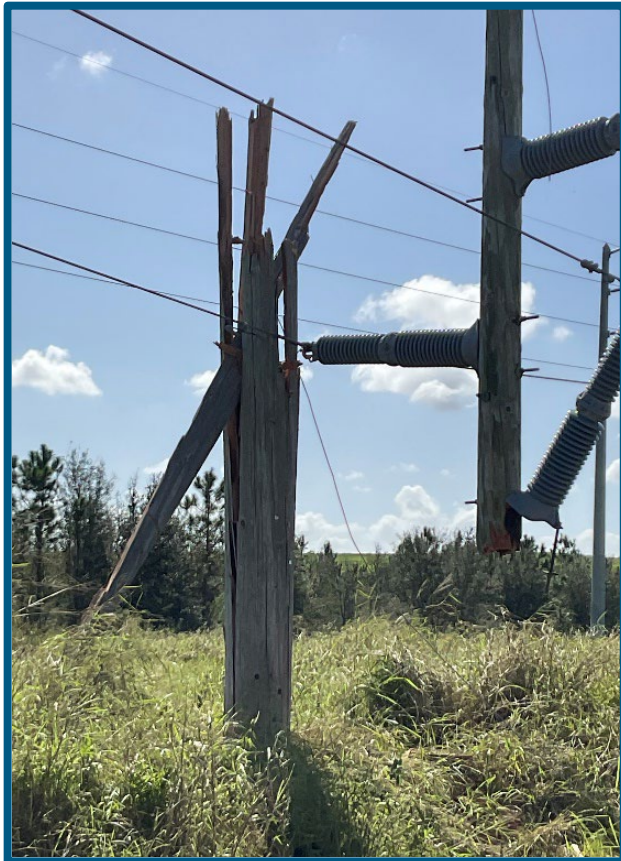
Figure 1: Broken Pole due to extreme weather event.
