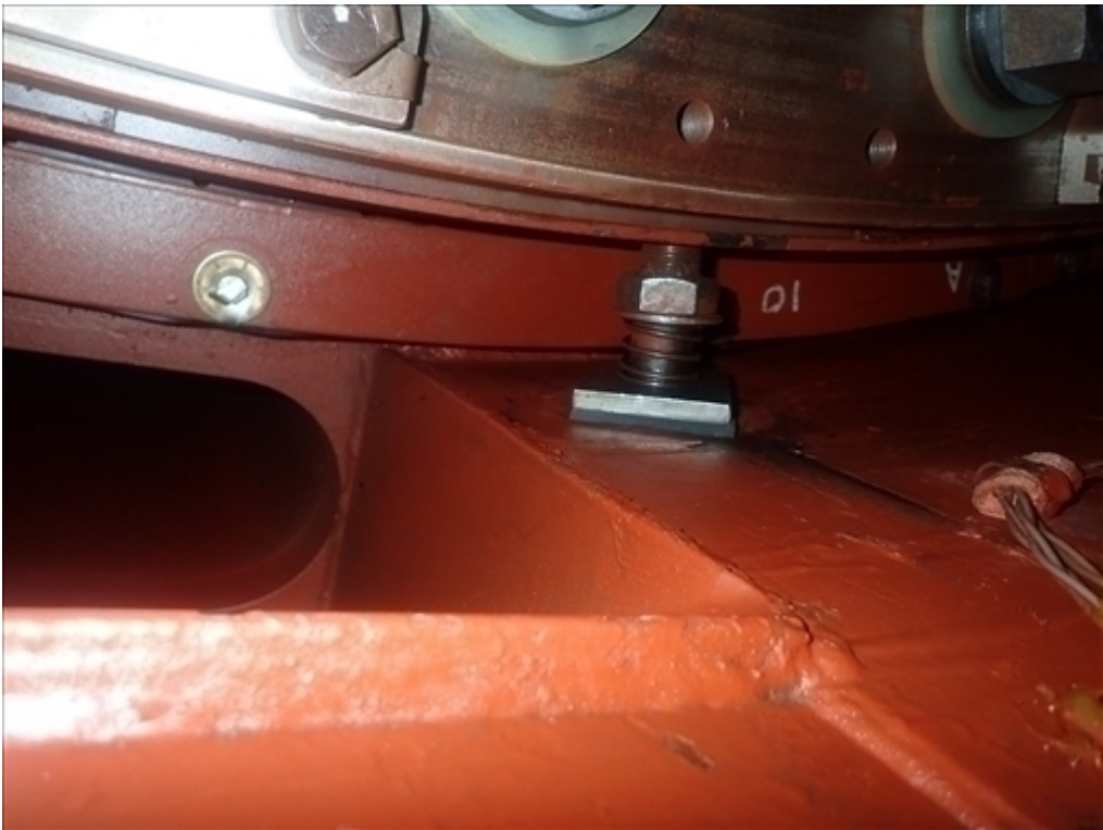
2.14 Turbine End Repaired End Shield Vent Tube Assembly
