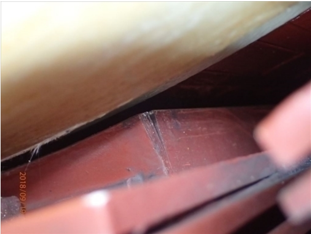
2.23 Exciter Stator Pole Iron Damage
