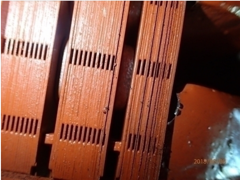
2.9 Typical Condition of Exciter and Turbine End Step Iron and Vents
