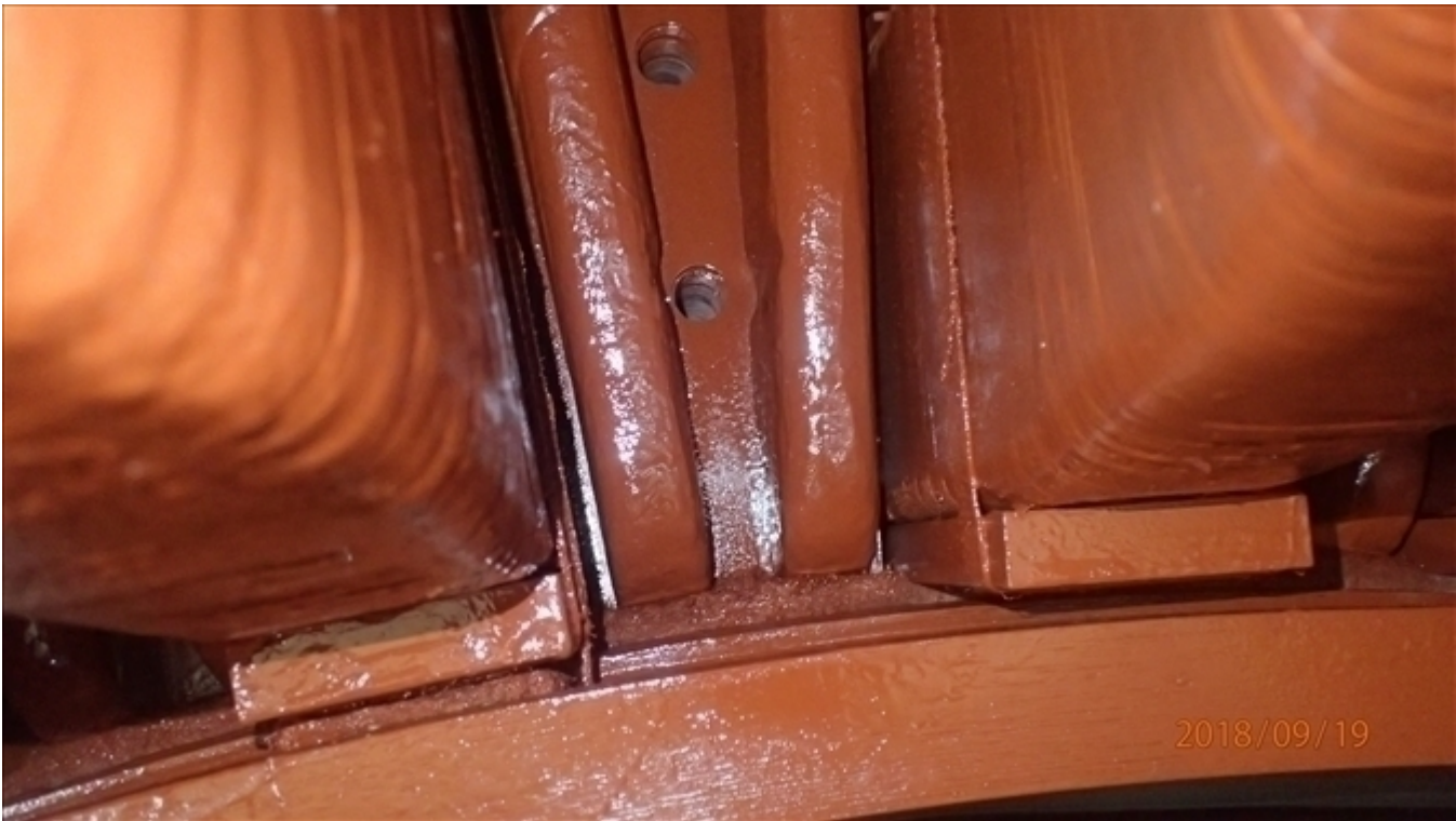
2.10 Typical Condition of Finger Plates After Painting
