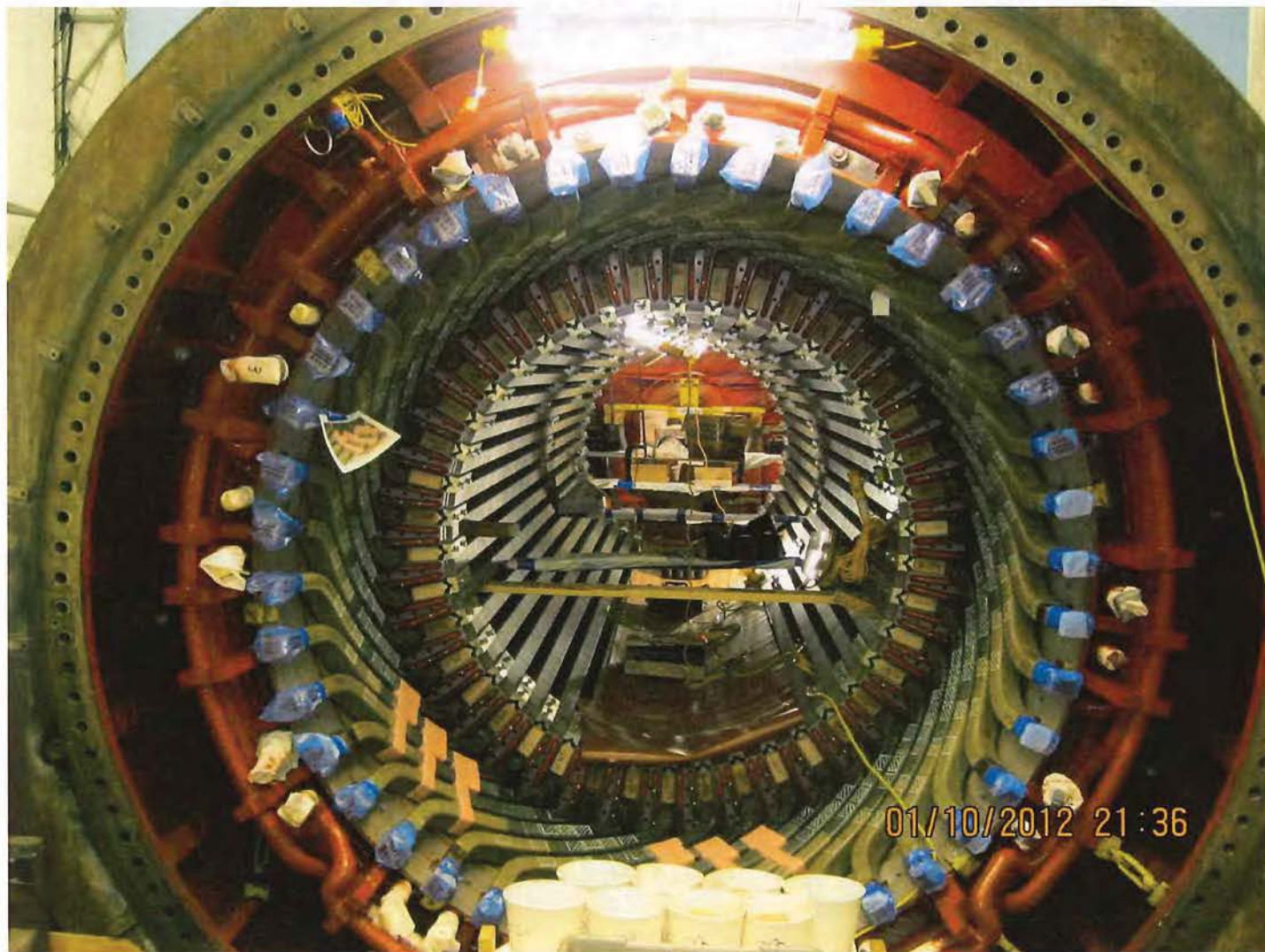
Figure 2 – Bottom Half-Coil installation
