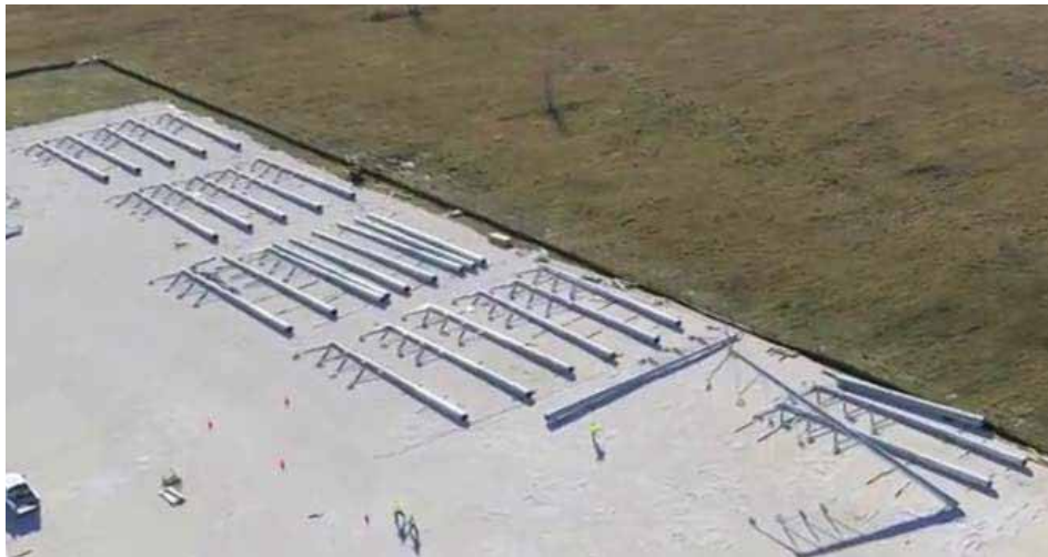
Framing the tops in the staging area
