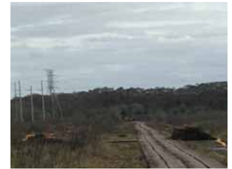
PHOTO OF TYPICAL LAYOUT OF WOOD & PLANK MATTING
