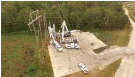
Typical Installation of a steel pole base
