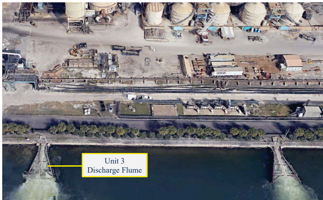
Figure 5 – Unit 3 and 4 Circulation Water Discharge Area
