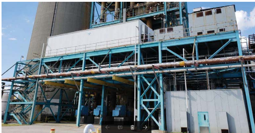
Figure 4 – Units 1 and 2 WFGD Electrical Building-to remain
