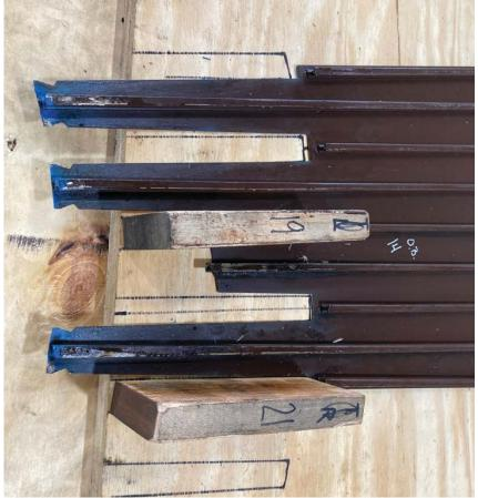
Loop Test After New Core Iron Installed
