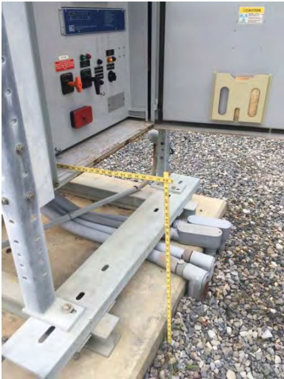
Feeder Breakers with water intrusion
