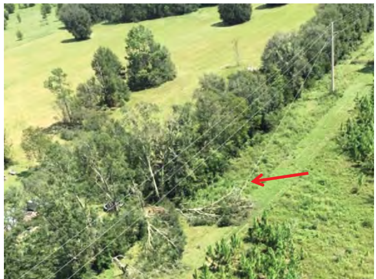
Structure 112R1 - Wire down due to vegetation
