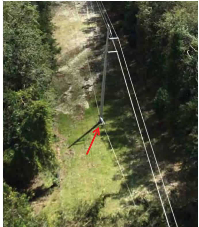
Structure 55R13A – Broken insulator
