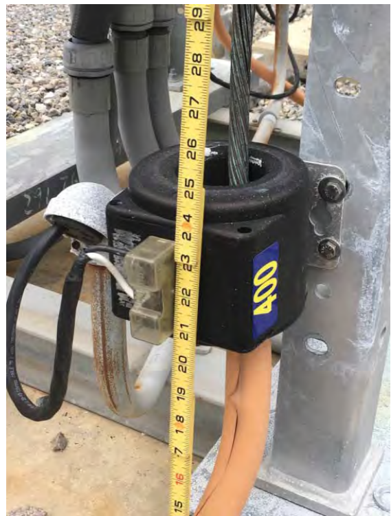
Fault bus CT's were submerged throughout entire substation
