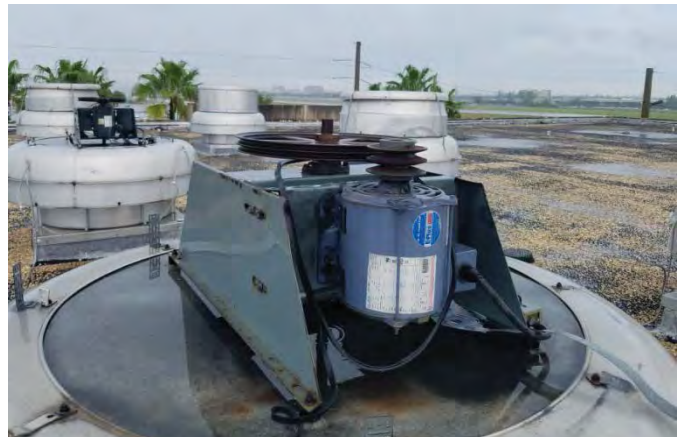
Watkins Substation – Roof Exhaust Fan
