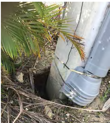
Base of leaning concrete pole
