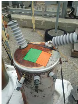
Broken bushings
