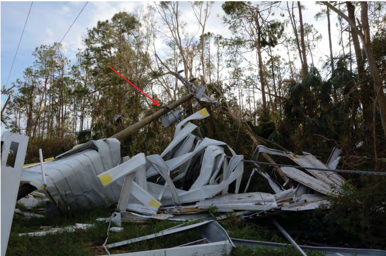
Pole down with transformer in West area due to trailer park debris
