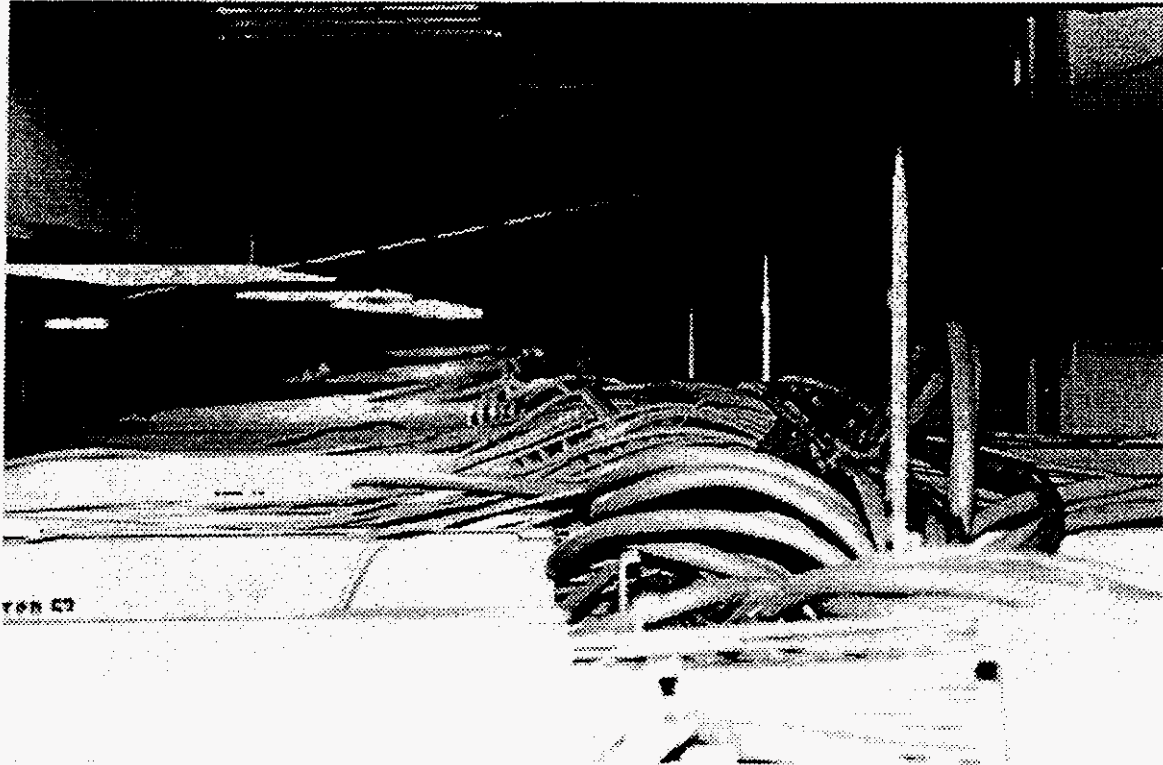
FIGURE 3: Cable trough congestion
