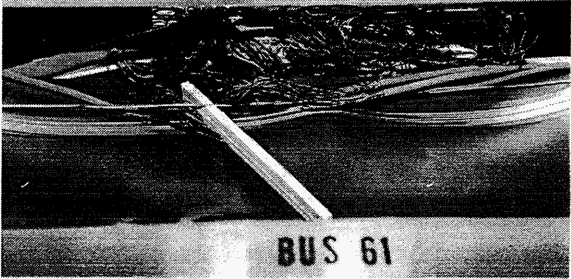
FIGURE 4: Detail of congestion caused by "in-trough" Y-splice.
