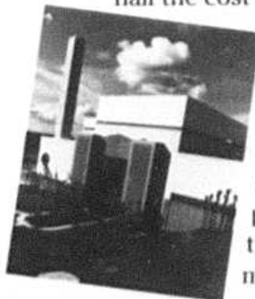
The new Lee County, Florida, waste-to-energy facility became the first in the nation to propose mercury abatement technology.
