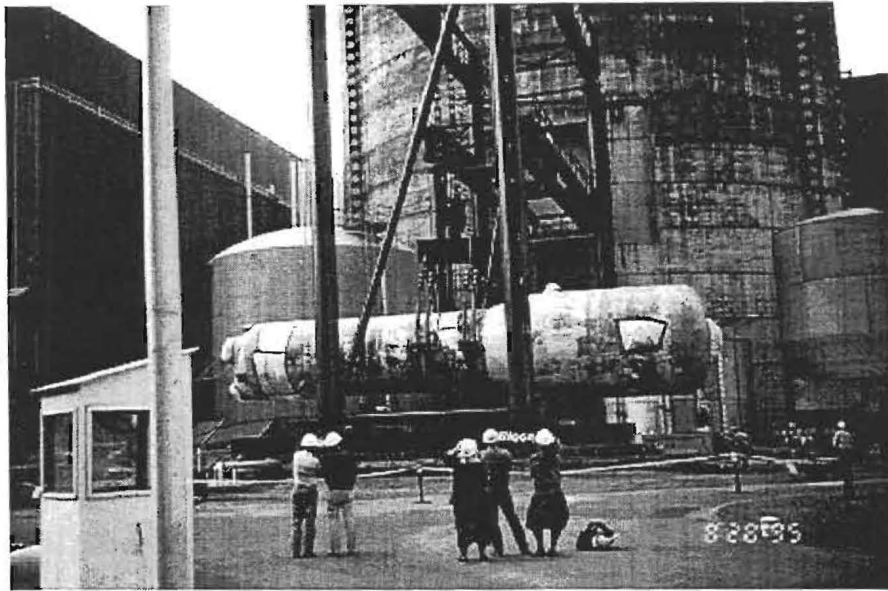
FIGURE 3.2 Removal of Steam Generator from Reactor Building
